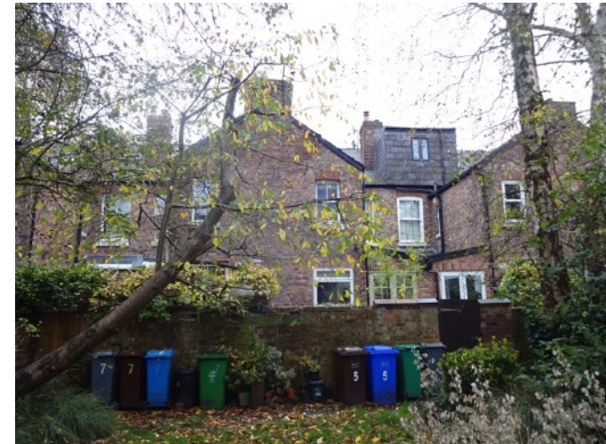
7.2 Existing rear dormer loft at 3 Stratford Avenue
