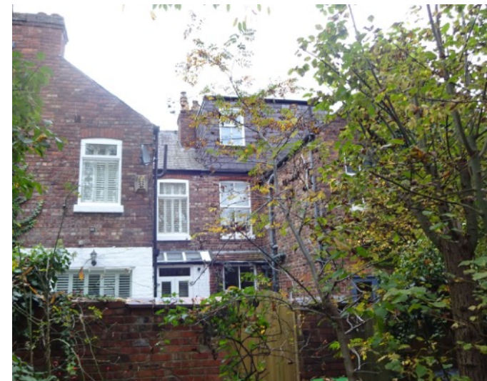
7.3 Existing rear dormer loft at 4 Northen Grove
