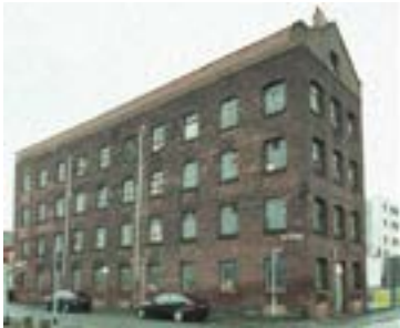
2. 8 Cable St (Grade II)
