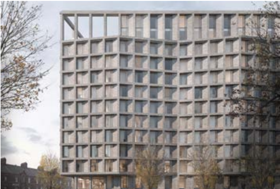
1. Bendix Street (13 storeys), under construction – Tim Groom Architects
