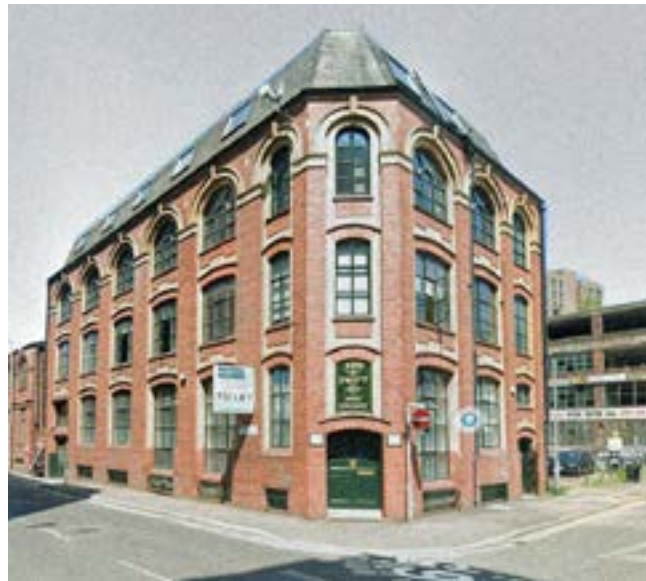
John Swift Building - adjacent to site
