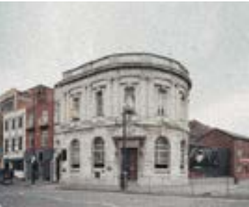
1. Former Midland Bank (Grade II)
