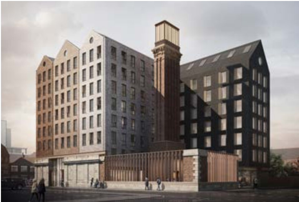
2. Goulden Street (9 storeys), under construction – Tim Groom Architects
