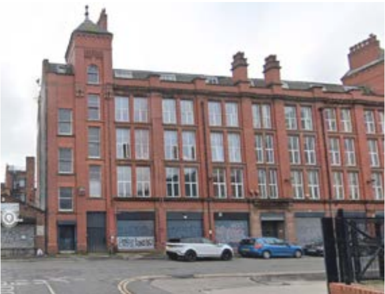
Cable Street - adjacent to site
