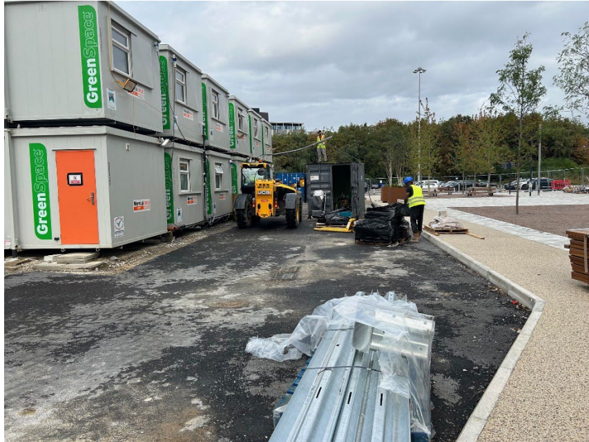
View west from northern site boundary
