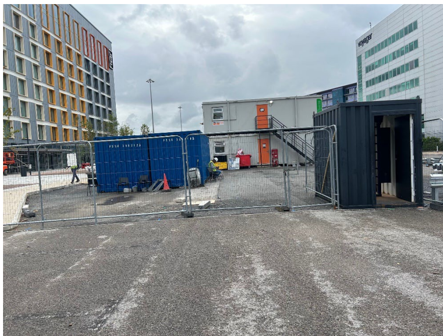
Material lay down / storage area in western portion of site
