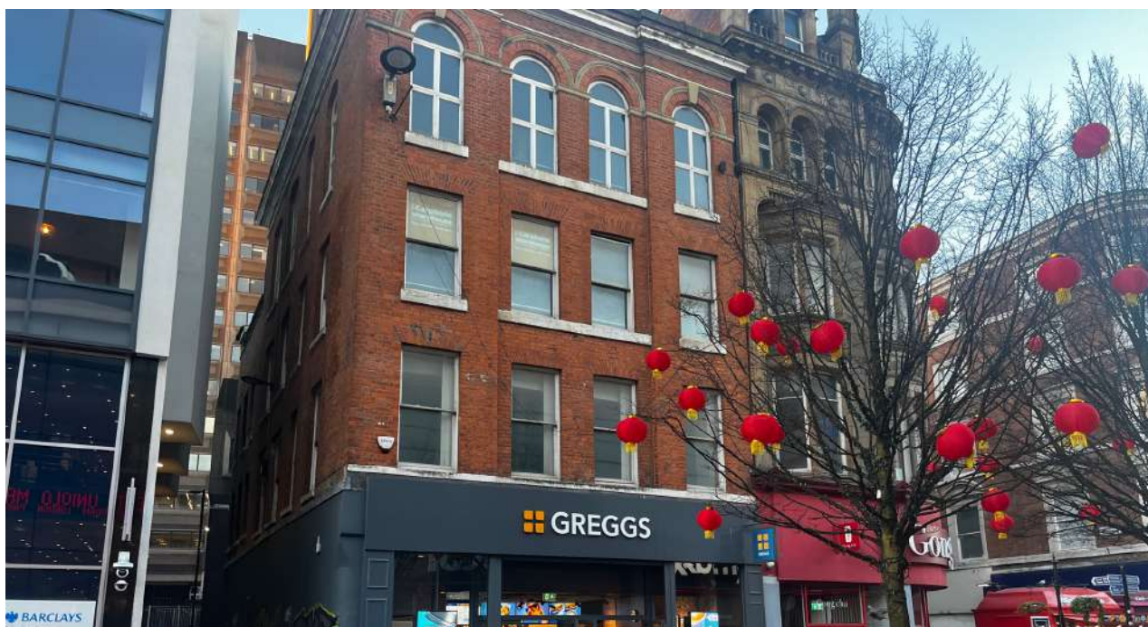
Photograph 2.2 : 82-84 Market Street – Upper Floors
