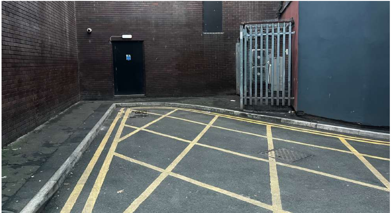
Photograph 2.7 : Sickle Street – Existing Rear of Building
