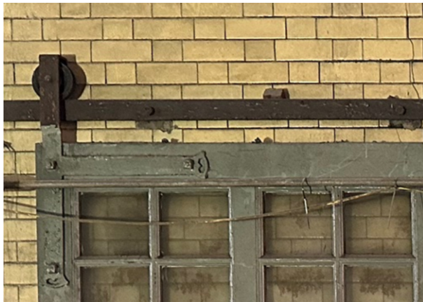
Door top hung on metal rail, fixed through masonry
