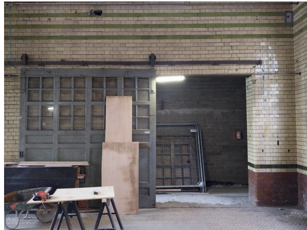
Photograph of the internal Ambulance Bay Door in situ
