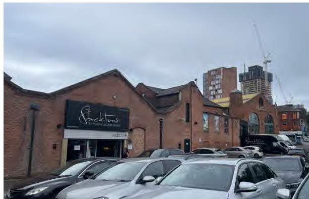
Figure 51 (left) and 52 (right), Building 2 (left) and Building 4 (former stable block): Images above depict the E elevation. Whilst the form of the buildings are largely unchanged, they have been subject to considerable alteration, including brick infill to window openings, new shop frontage and signage.
