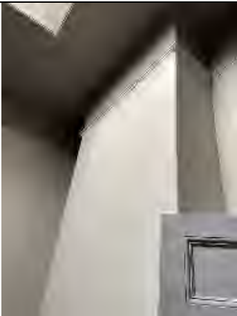
Figure 93: Original chimney breast, skirting and cornice survives.
