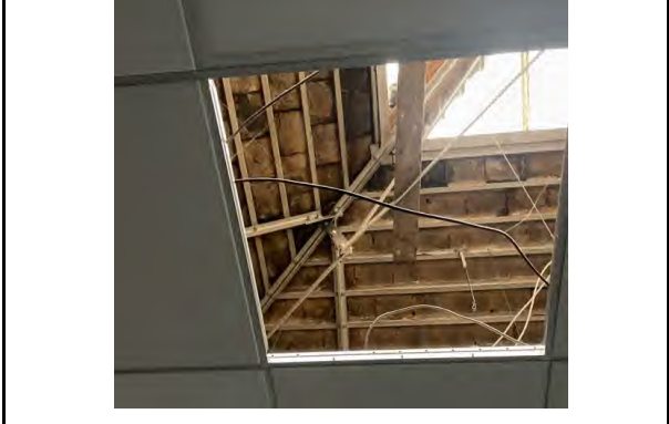
Figure 64: Original ceiling tile and trusses to warehouse visible through modern suspended ceiling.
