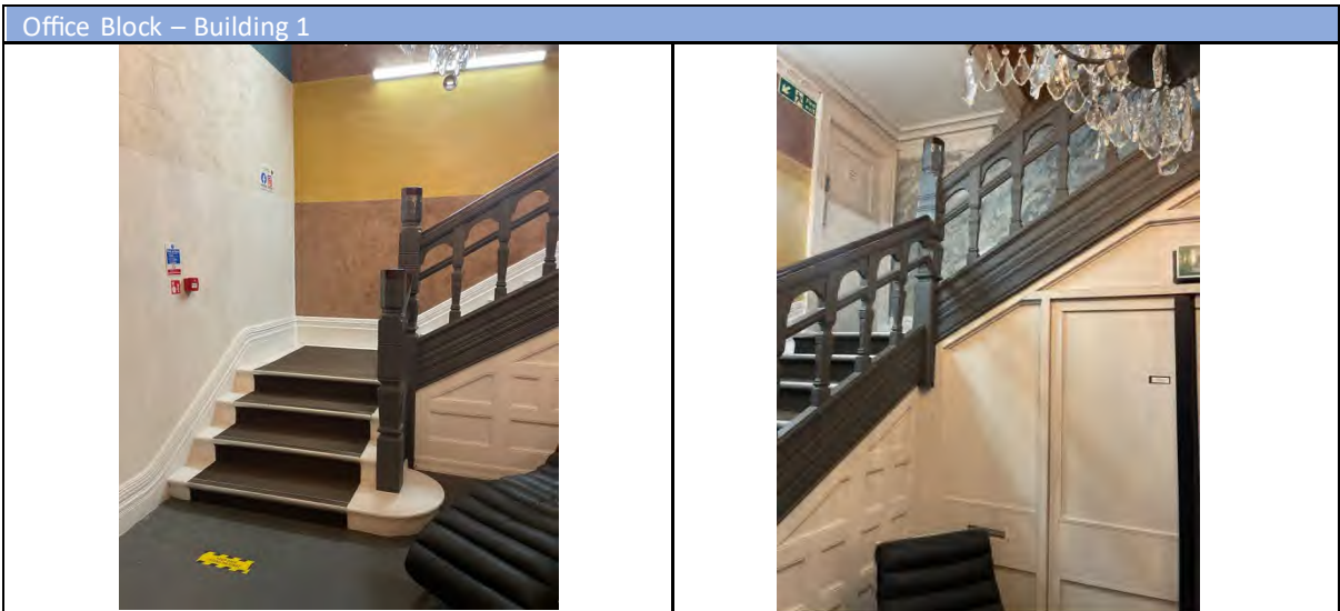
Figure 75 and 76: Original staircase c.1900, with original skirting, panelling and balustrade. Modern infill to far right, enclosing the former entrance from Store Street.
