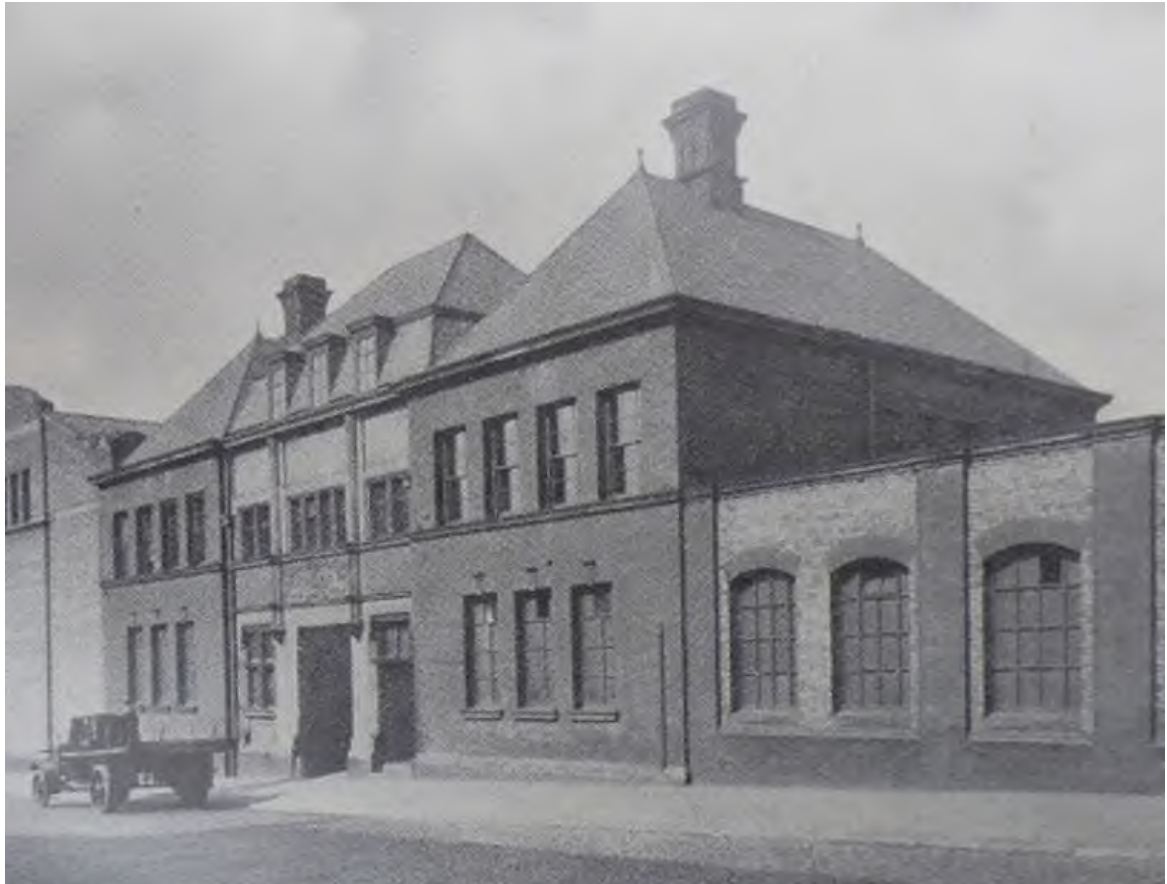
Figure 33: Office Block to Store Street, pictured c.1926. Note, the central block differs from the 1899 plan, with the sandstone 2 ½ storey range to the centre. Source: Dunkerley & Co. store booklet.
