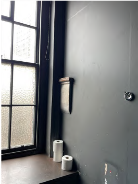
Figure 107: Original tobins vent and sash window feature within the WC space.
