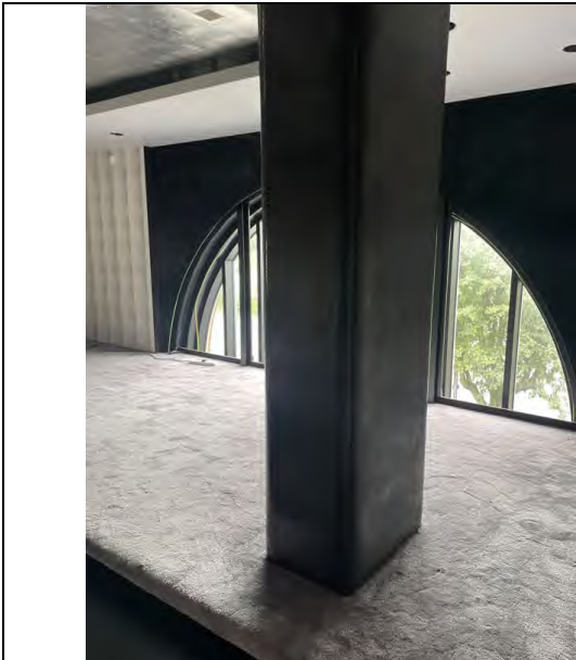
Figure 127: Modern floor to former double height space, modern column arrangement.
