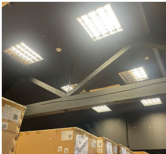
Figure 74: Original double pitched truss arrangement.
