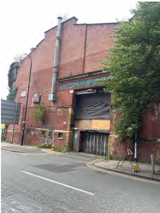
Figure 55: Original opening to former girder warehouse. Note, this building is not within the Planning Site boundary, but forms the immediate setting of the site.
