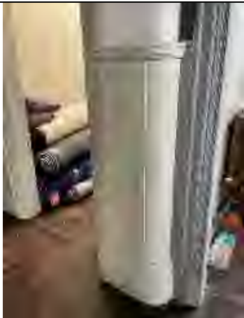
Figure 97: Simple plaster moulding to dado height, with banded detail and deep skirting.
