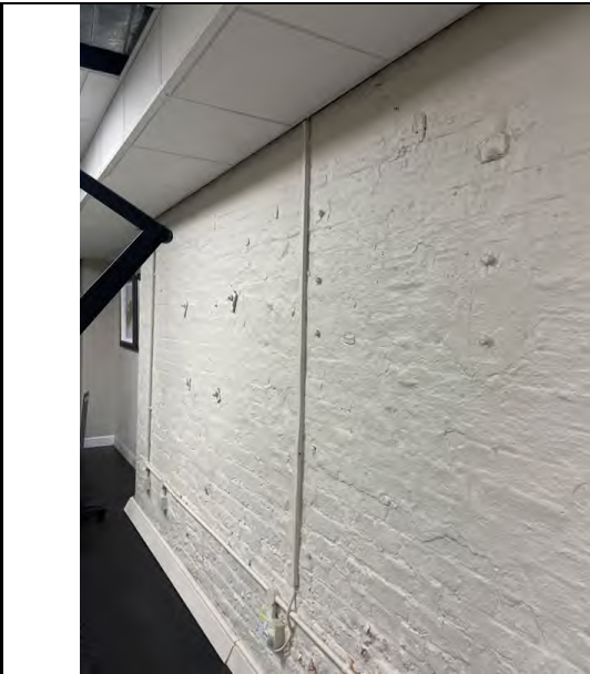
Figure 128: Original brick wall to ground floor space. Modern suspended ceilings and flooring throughout.
