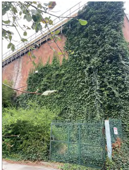
Figure 56: West elevation to girder warehouse. Note, this building is not within the Planning Site boundary, but forms the immediate setting of the site.
