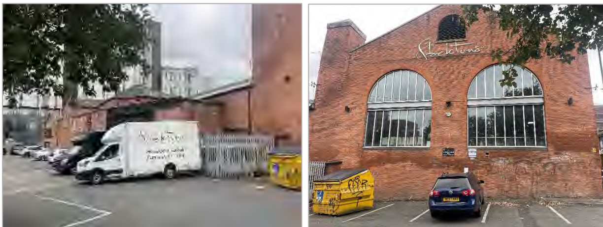
Figure 1: Stocktons entrance, north elevation. Figure 2: 1836-1850s warehouse, now a showroom. Source: SLHA site visit, August 2024.
