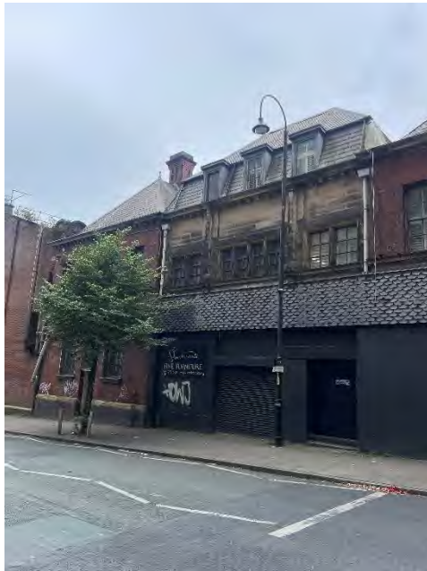
Figure 49 (left) and 50 (right): Building 1 (Office Block). Store Street elevation, south. Built early 1900s. Two equal red brick wings feature, of 2-storeys in height, with a slate roof and central chimney stack. A central section built of stone with a mansard roof and three dormer windows (non-original), with three bays at first floor, featuring original metal framed windows. The façade has been altered with fish scale banding between ground and first floor level.
