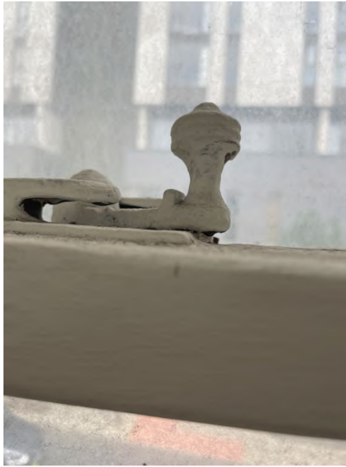
Figure 115: Original window latch.
