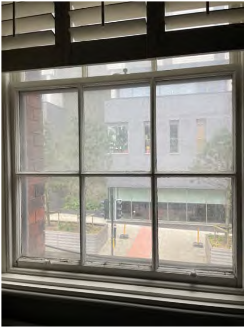
Figure 114: Original sash window, detail.
