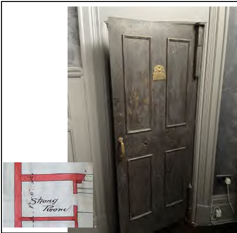
Figure 90: Original Strong Room door with brass ironmongery and panelling detail.
