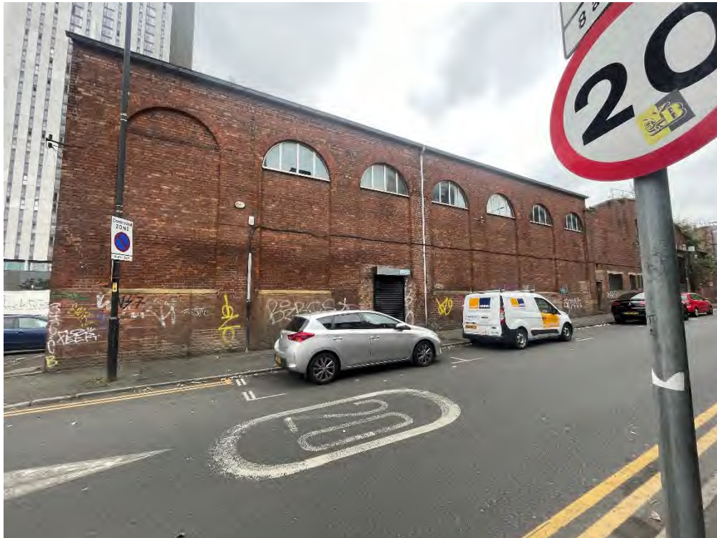
Figure 123: Mid-19 th century warehouse / former riveting workshop. North elevation to Ducie Street. Seven equal bays with recessed arch detail. Six with later windows installed to arch. Modern roller shutter door.
