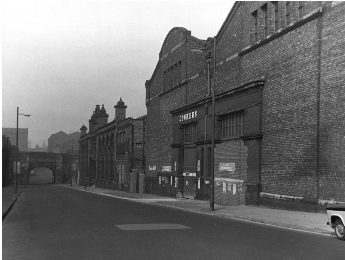
Figure 18: Historic image, 1966. Store Street, looking south-west, with Store Street aqueduct visible to far left. The expansive Girder Warehouse, consisting of two equal bays is visible to the far left, this originally formed part of the C. C. Dunkerley Site, but was later used by 'Lookers' car dealership. Source: Manchester Image archive, ref: M05942.
