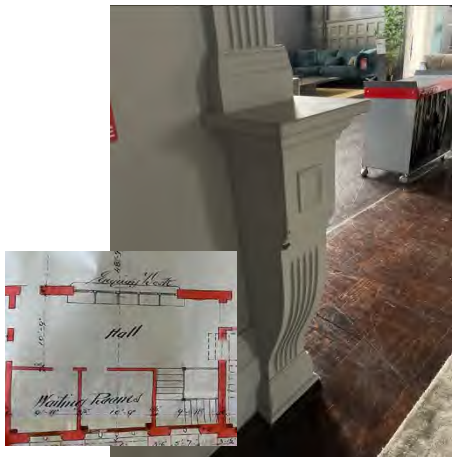
Figure 84: Original timber wall bracket with fluted detail, historically enclosed each side to the waiting desk.
