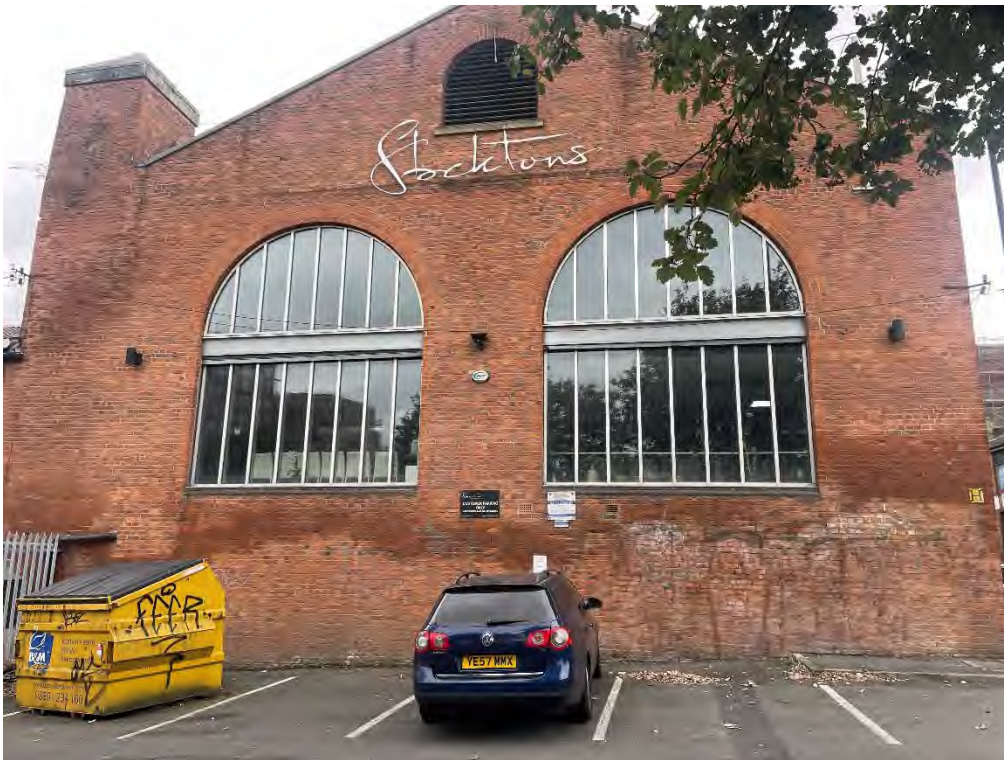
Figure 122: Mid-19 th century warehouse, built c.1836 -1850 of red brick in English bond. Later windows installed within two arched openings. Modern 'Stocktons' signage above. Original chimney base visible to left of image, the stack has been removed.
