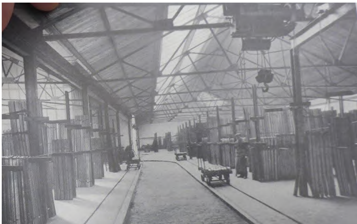
Figure 37: Packing Hoop Warehouse, pictured c.1926. Source: Dunkerley & Co. store booklet.
