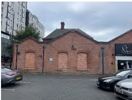
Figure 51 (left) and 52 (right), Building 2 (left) and Building 4 (former stable block): Images above depict the E elevation. Whilst the form of the buildings are largely unchanged, they have been subject to considerable alteration, including brick infill to window openings, new shop frontage and signage.
