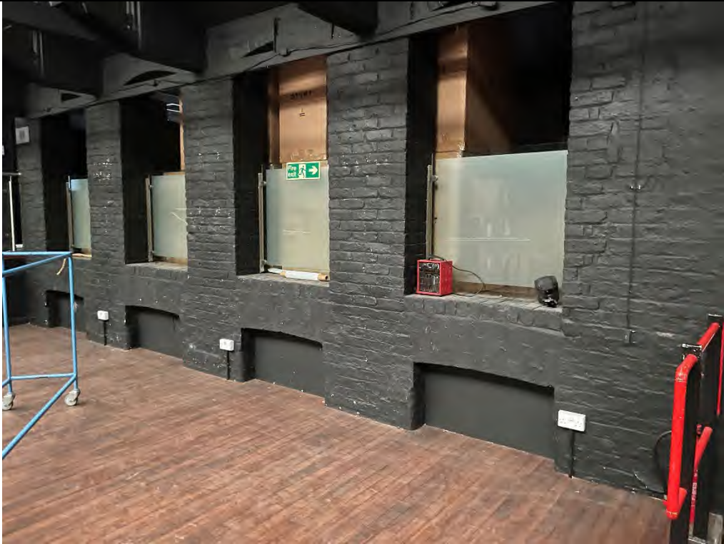
Figure 72: Mid-19 th century warehouse building. Former external wall (south). Modern raised floor to bar warehouse. Modern infill to windows and modern glazing.
