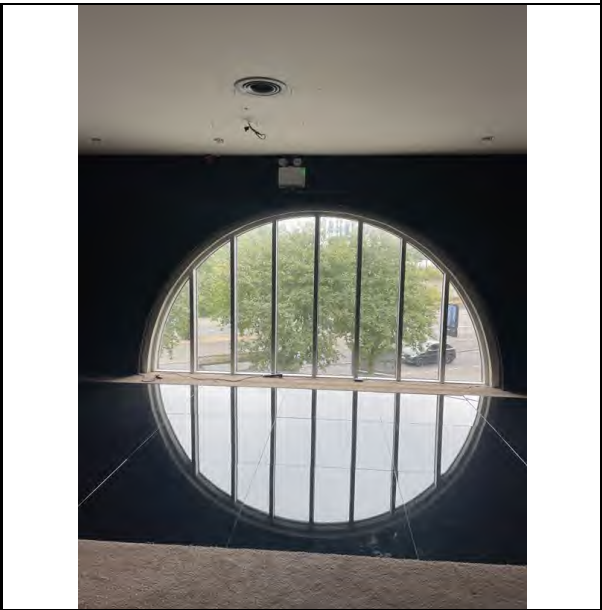
Figure 126: Later window insertion to arch. East elevation, fronting Great Ancoats Street.
