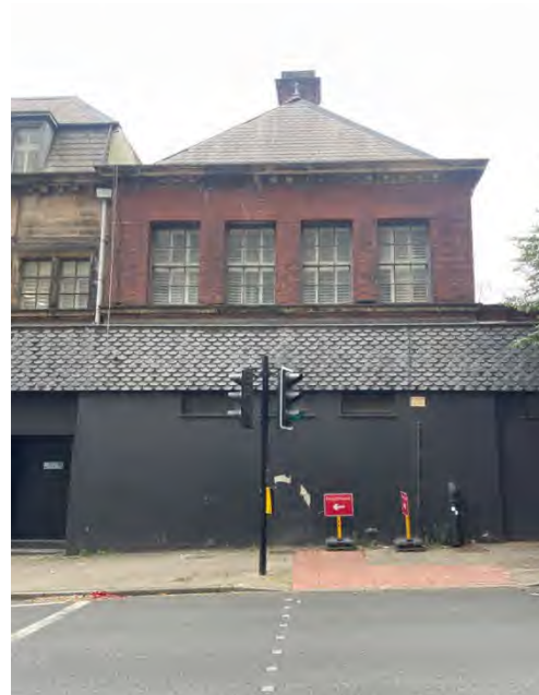
Figure 49 (left) and 50 (right): Building 1 (Office Block). Store Street elevation, south. Built early 1900s. Two equal red brick wings feature, of 2-storeys in height, with a slate roof and central chimney stack. A central section built of stone with a mansard roof and three dormer windows (non-original), with three bays at first floor, featuring original metal framed windows. The façade has been altered with fish scale banding between ground and first floor level.
