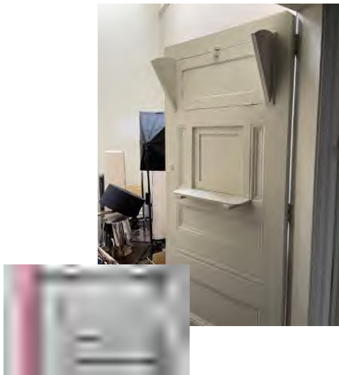
Figure 94: Original timber door with casement opening and central hatch (Typewriter room).
