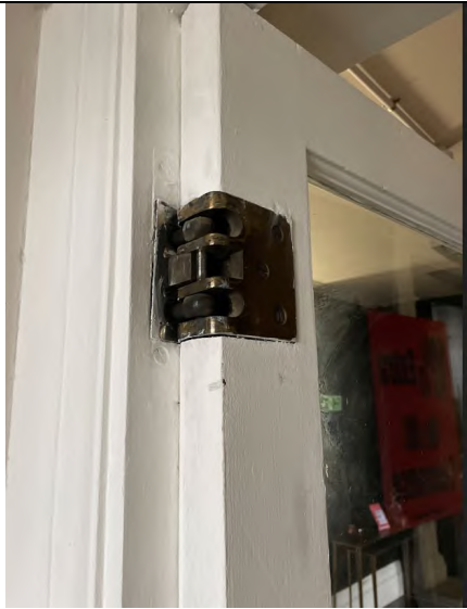
Figure 117: Brass hinge to original door (later glazing).
