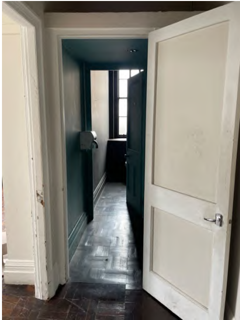
Figure 106: Single toilet / WC area, later addition – modern door.
