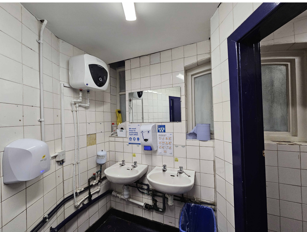
08 - Existing Driver's WCs
