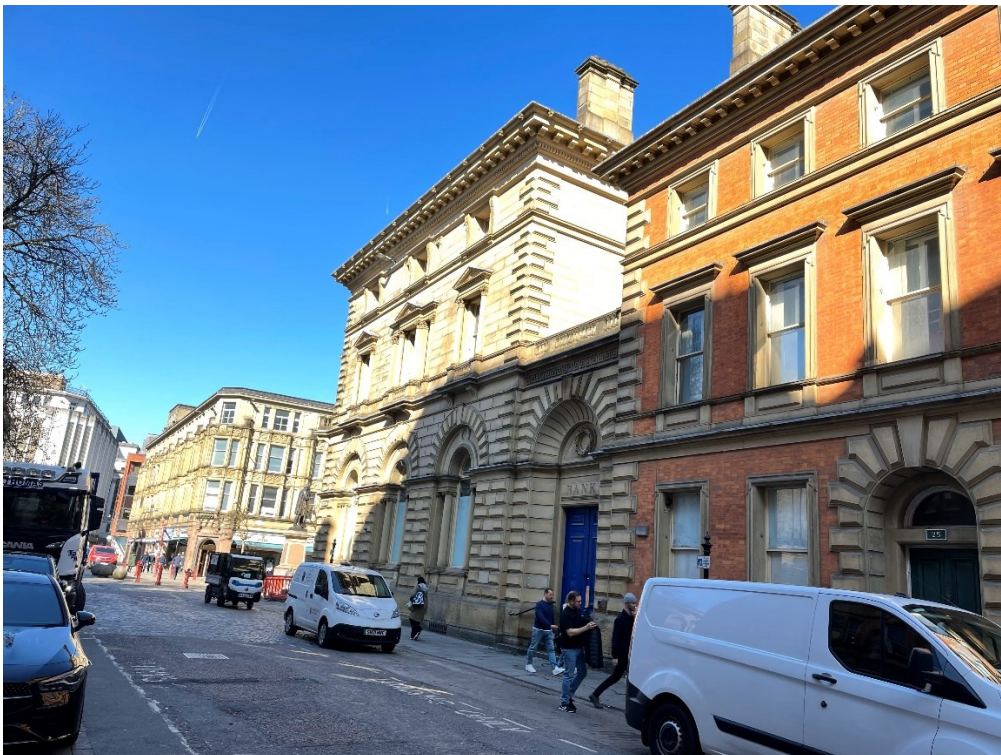
Figure 2 - Photograph of 25 St Anns Street from St Anns Street
