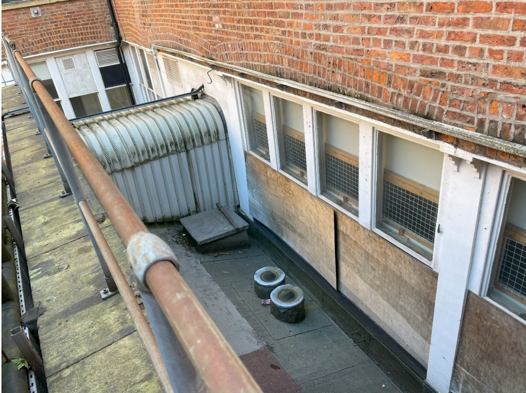
Figure 1 - Stepped access tunnel photograph from the roof
