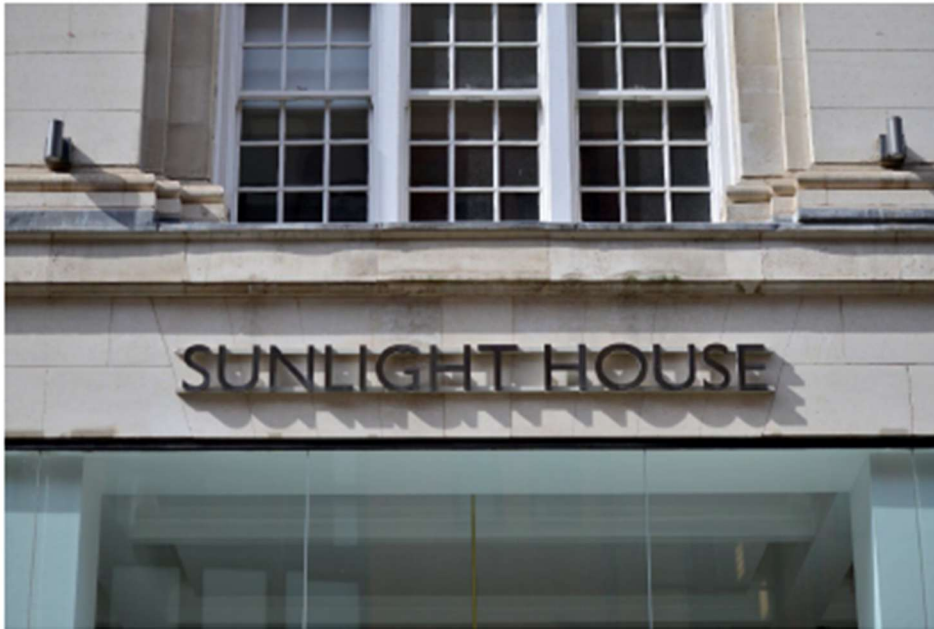
Existing signage to main entrance on Little Quay Street
