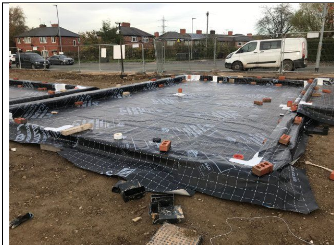
Evidence of gas membrane installed across Plot 6.
