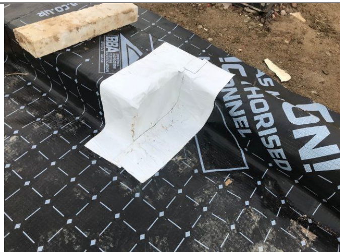
Example of overlapping and sealing of gas membrane appropriately sealed at joints in Plot 6.
