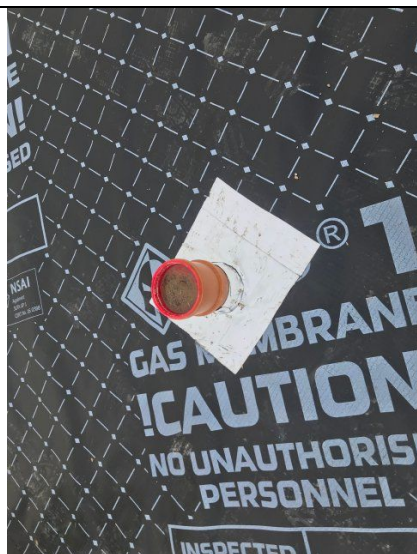
Evidence of top hats and sealing at service entry points in Plot 6.
