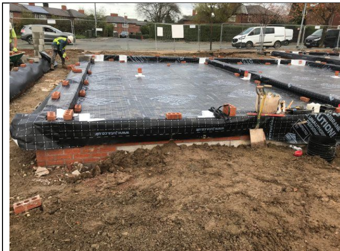
Evidence of gas membrane installed across Plot 8.
