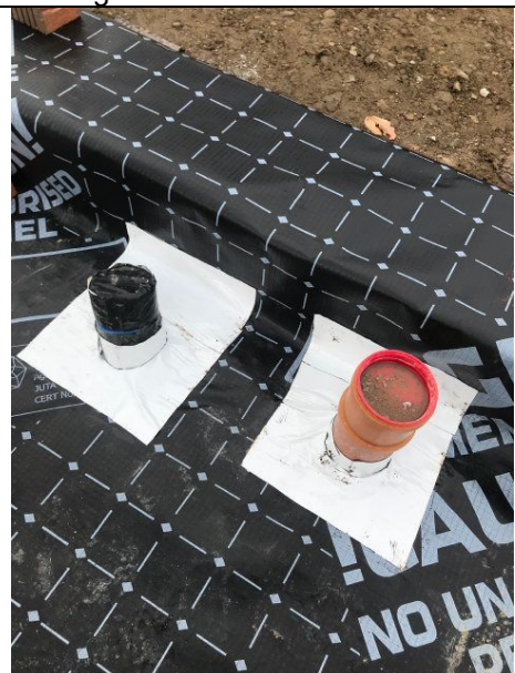
Evidence of top hats and sealing at service entry points in Plot 5.
