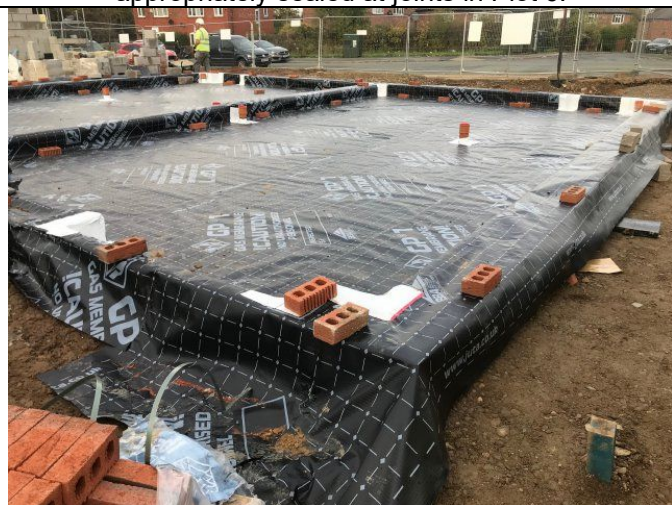
Example of overlapping and sealing of gas membrane appropriately sealed at joints in Plot 6.
