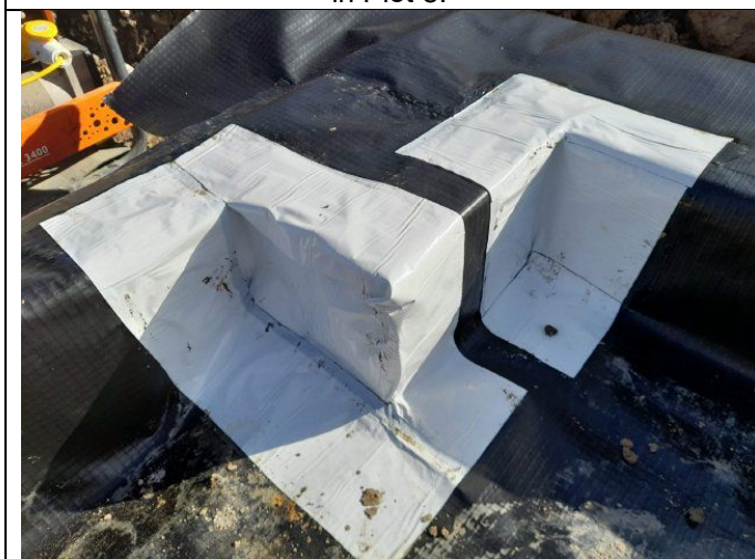
Example of overlapping and sealing of gas membrane appropriately sealed at joints in Plot 9.
