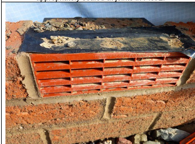
Evidence of installation of air bricks in Plot 2.
