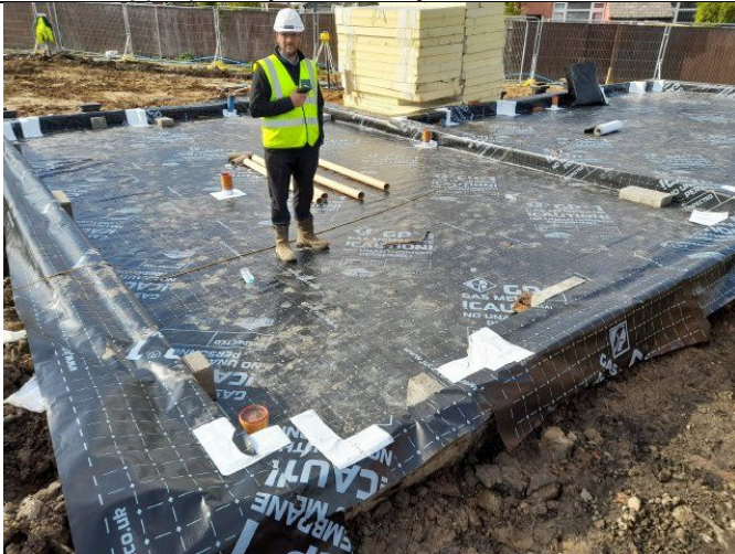
Evidence of gas membrane installed across Plots 11 and 12.
