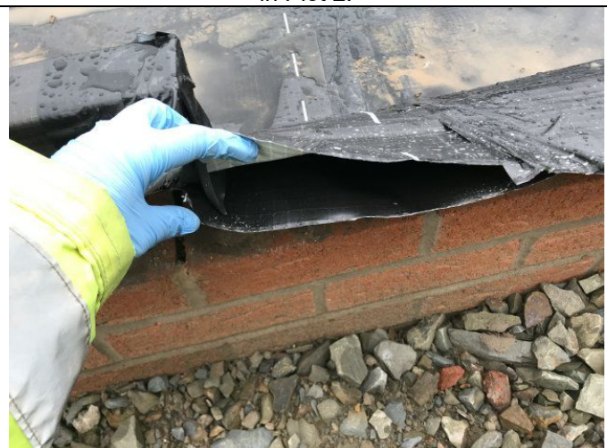
Example of overlapping and sealing of gas membrane appropriately sealed at joints in Plot 3.
