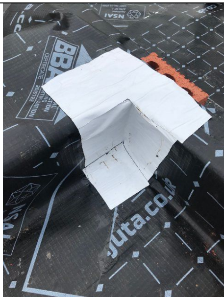
Example of overlapping and sealing of gas membrane appropriately sealed at joints in Plot 5.
