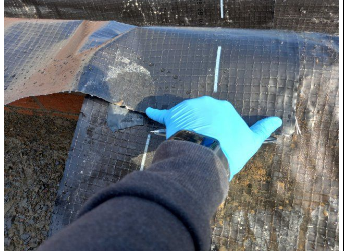
Example of overlapping and sealing of gas membrane appropriately sealed at joints in Plot 1.
