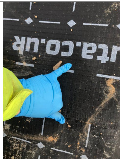
Example of overlapping and sealing of gas membrane appropriately sealed at joints in Plot 8.
