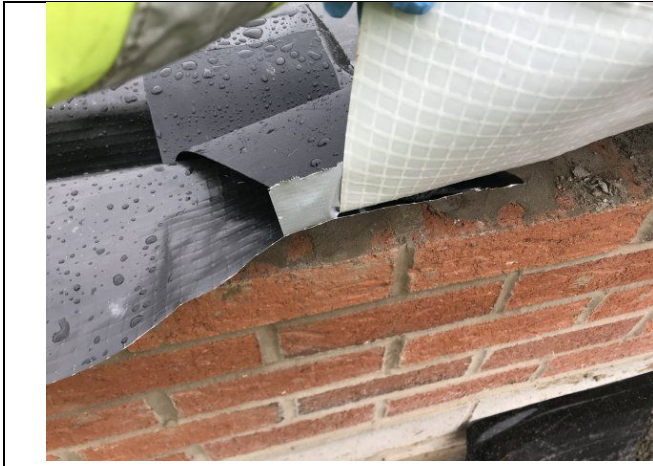
Example of overlapping and sealing of gas membrane appropriately sealed at joints in Plot 4.
