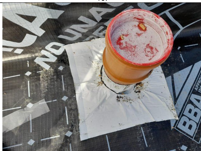
Evidence of top hats and sealing at service entry points in Plot 9.
