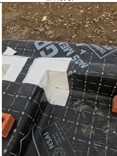
Example of overlapping and sealing of gas membrane appropriately sealed at joints in Plot 7.
