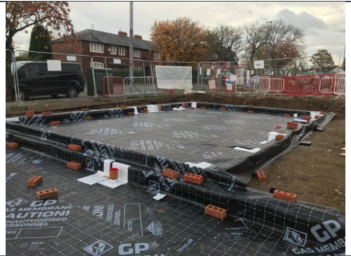
Evidence of gas membrane installed across Plot 5.
