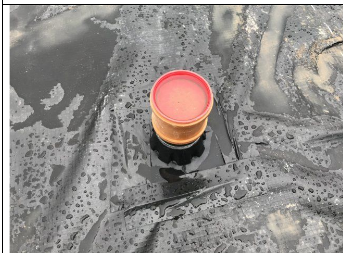
Evidence of top hats and sealing at service entry points in Plot 3.
