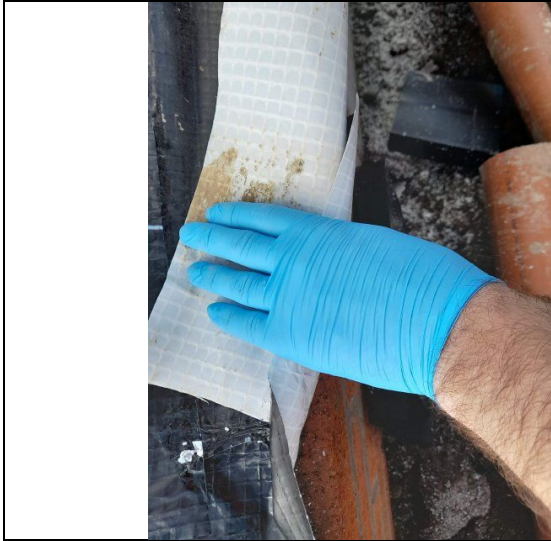
Example of overlapping and sealing of gas membrane appropriately sealed at joints in Plot 10.
