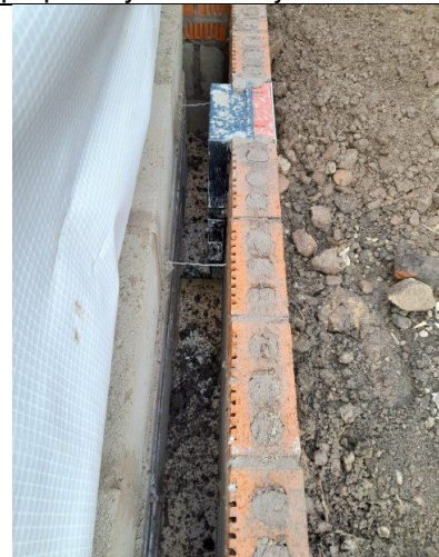
Evidence of installation of air bricks in Plot 11.
