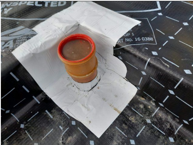
Evidence of top hats and sealing at service entry points in Plot 11.
