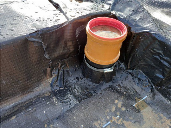
Evidence of top hats and sealing at service entry points in Plot 1.
