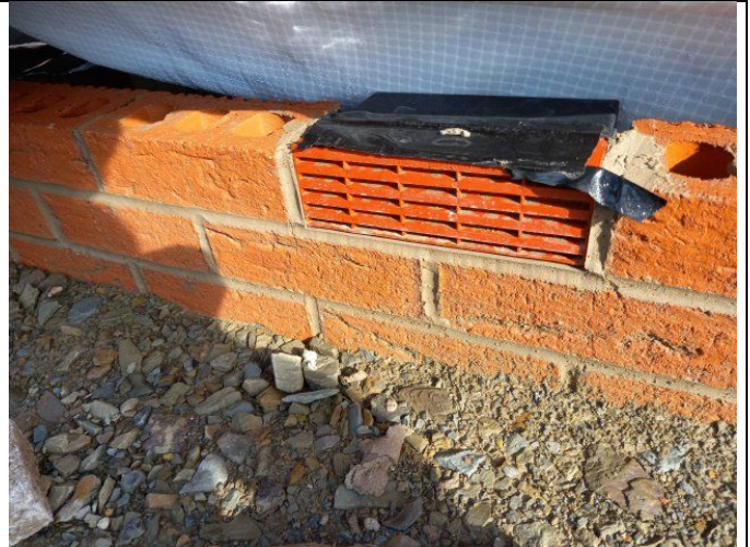
Evidence of installation of air bricks in Plot 1.
