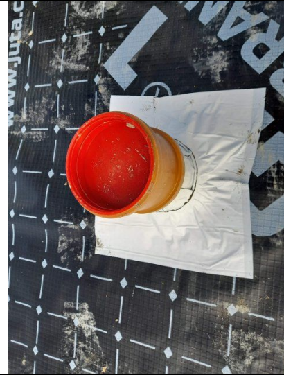
Evidence of top hats and sealing at service entry points in Plot 10.
