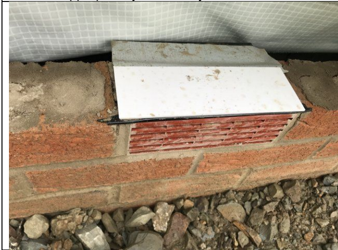
Evidence of installation of air bricks in Plot 4.
