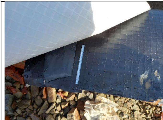
Example of overlapping and sealing of gas membrane appropriately sealed at joints in Plot 2.
