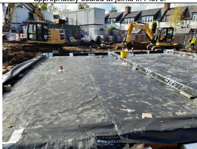
Example of overlapping and sealing of gas membrane appropriately sealed at joints in Plot 8.
