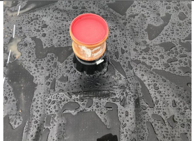
Evidence of top hats and sealing at service entry points in Plot 4.
