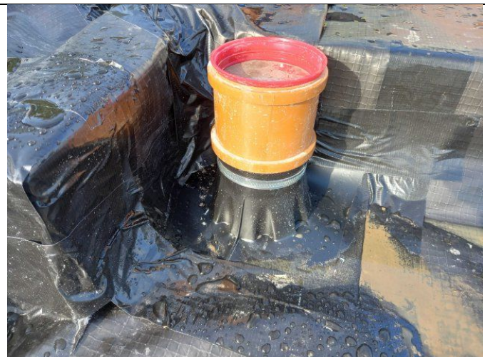
Evidence of top hats and sealing at service entry points in Plot 2.
