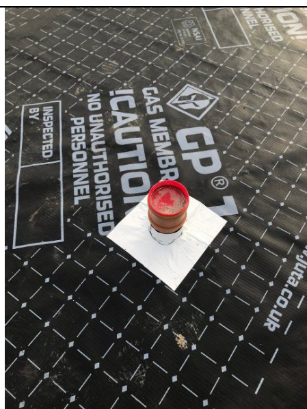
Evidence of top hats and sealing at service entry points in Plot 8.
