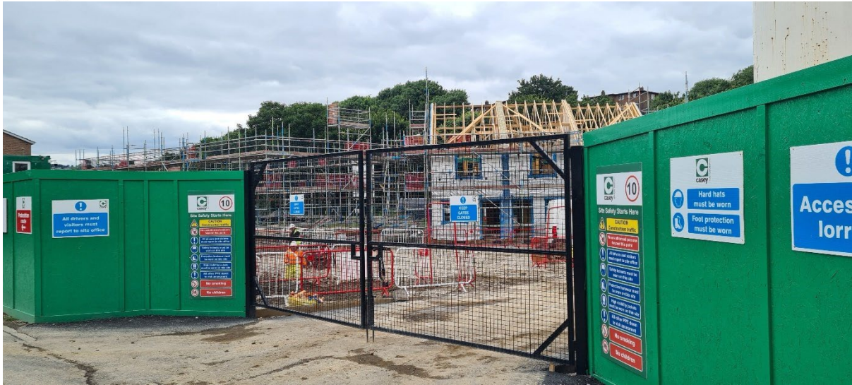
Hoarding and Heras securing site. Fig 2
