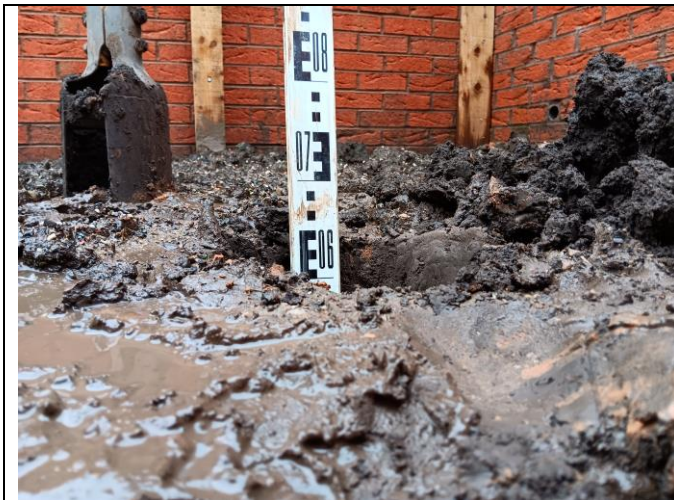
Photograph 6: Evidence of suitably chemically validated topsoil with a minimum of 150mm growing medium in garden areas (Plot 6) over natural strata.
