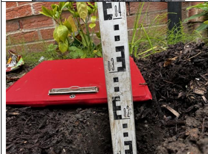
Photograph 8: Evidence of suitably chemically validated topsoil with a minimum of 150mm growing medium in front garden area (Plot 6) over natural strata.
