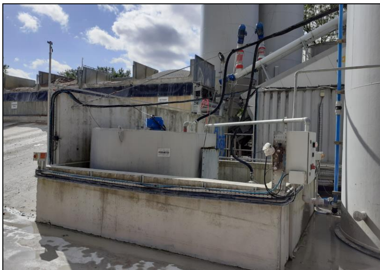
Figure 4.4 – Micro Silica storage (source: Heidelberg Materials)
