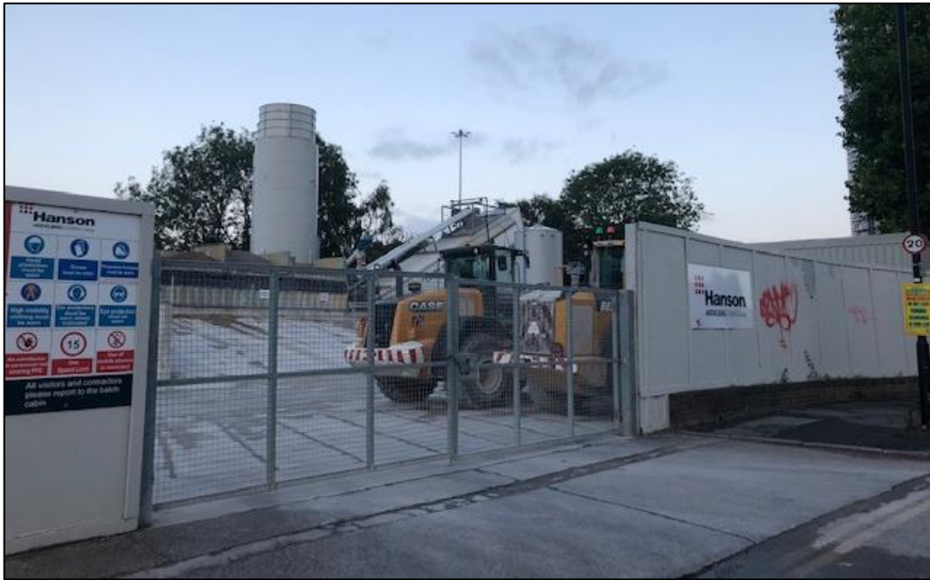
Figure 4.2: Plot D Concrete Batching Plant (source: Renaker Build Ltd)
