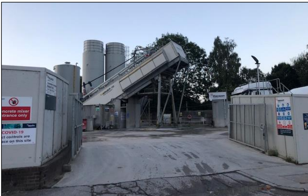
Figure 4.1: Plot D Concrete Batching Plant (source: Renaker Build Ltd)
