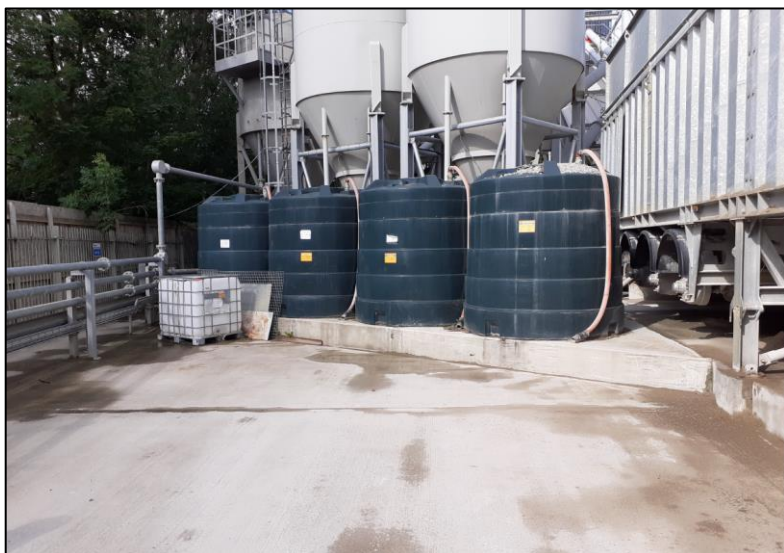
Figure 4.3 - Admixtures tanks (source: Heidelberg Materials)
