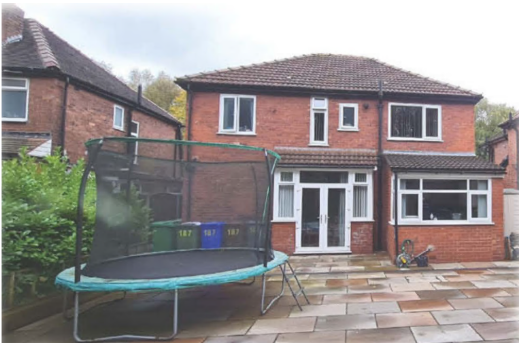
Image 3 Photograph of the rear elevation provided by the applicant as part of the submitted drawings
