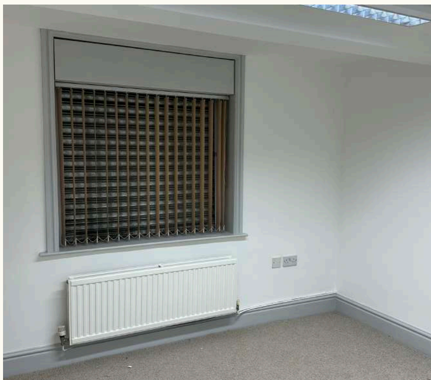
REF 16: BASEMENT WINDOWS
