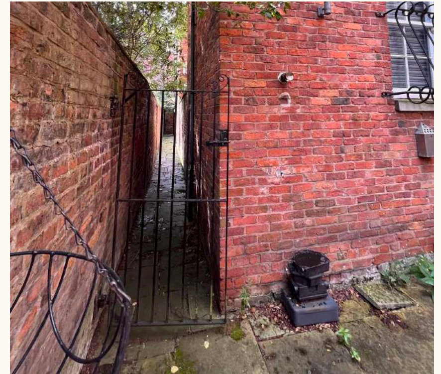
REF 3: REAR ACCESS TO THE PROPERTY
