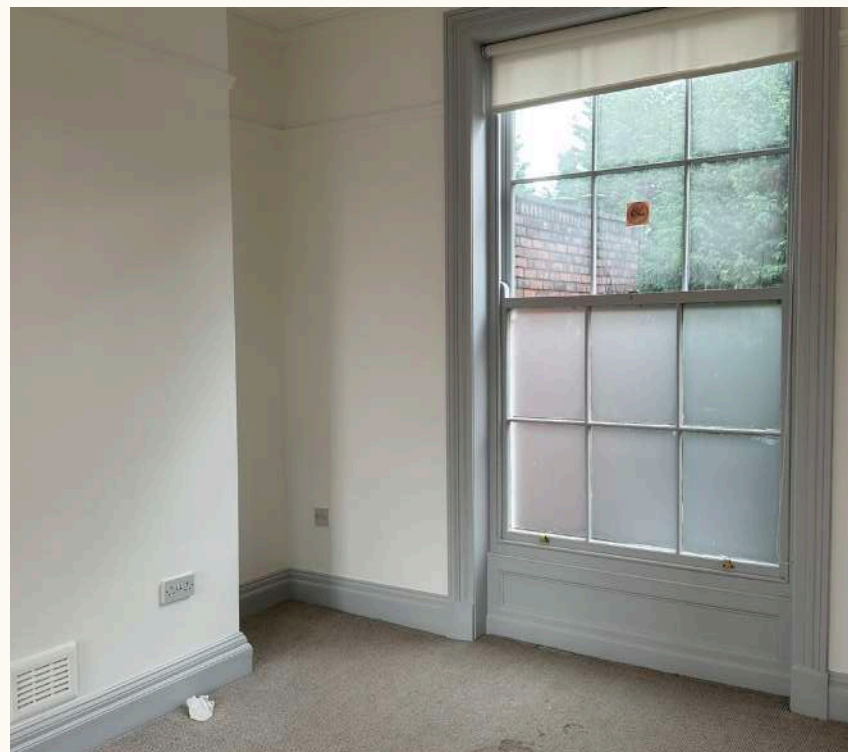
REF 11: FIRST FLOOR WINDOW CONDITION
