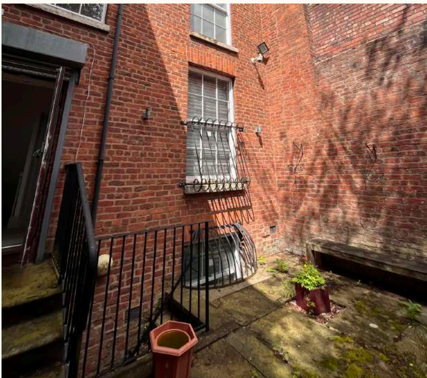
REF 4: ENCLOSED REAR YARD WITH ACCESS TO THE BASEMENT LEVELS
