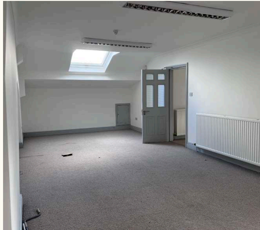
REF 8: SECOND FLOOR INTERIOR ROOM FINISHES
