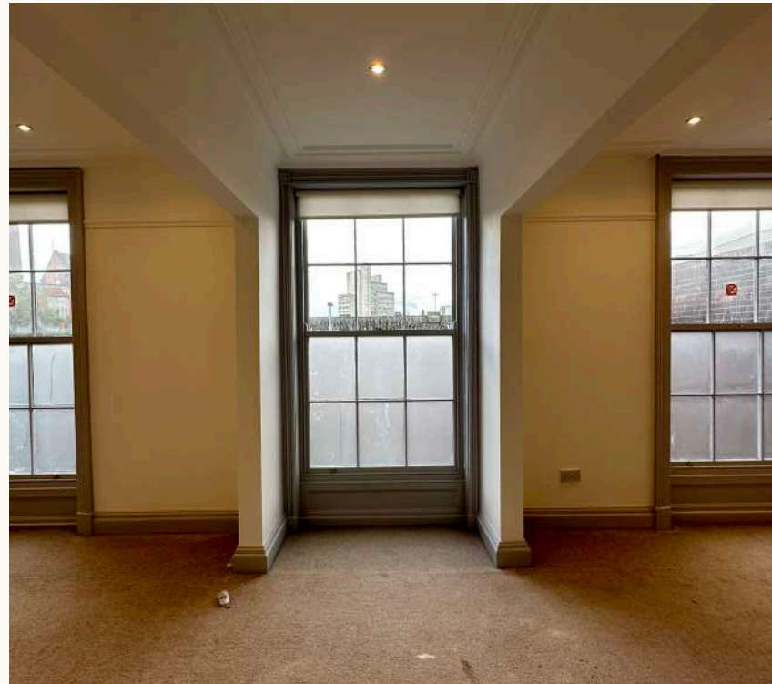
REF 14: FIRST FLOOR FRONT WINDOWS
