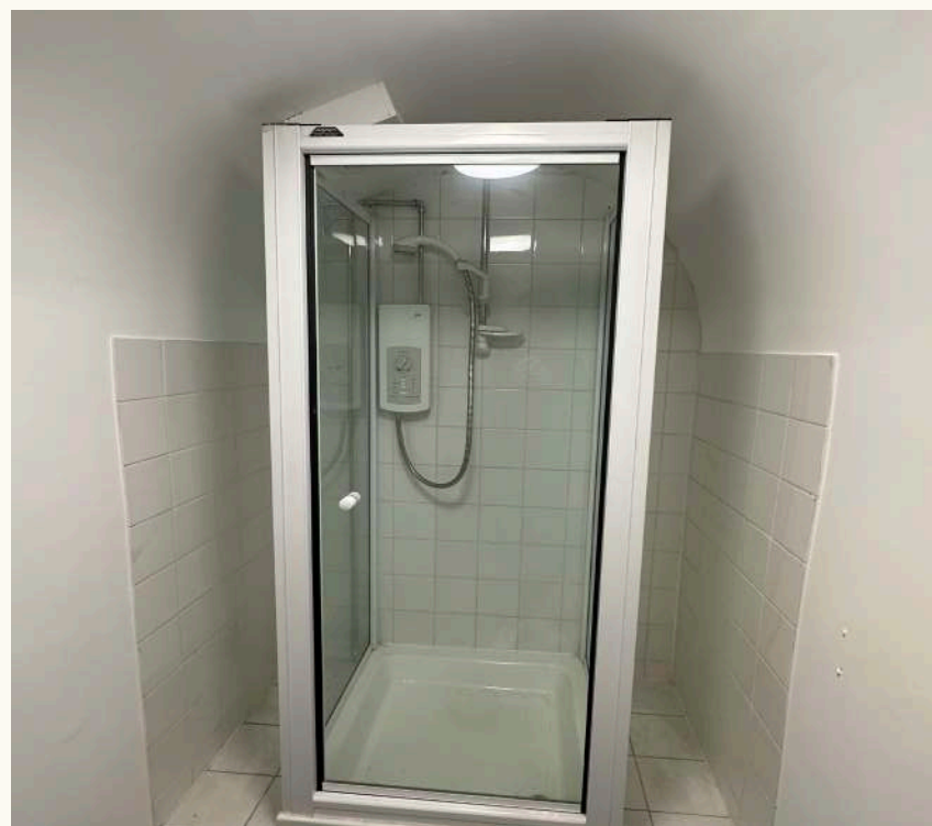
REF 17: BASEMENT VAULTED CEILING SHOWER
