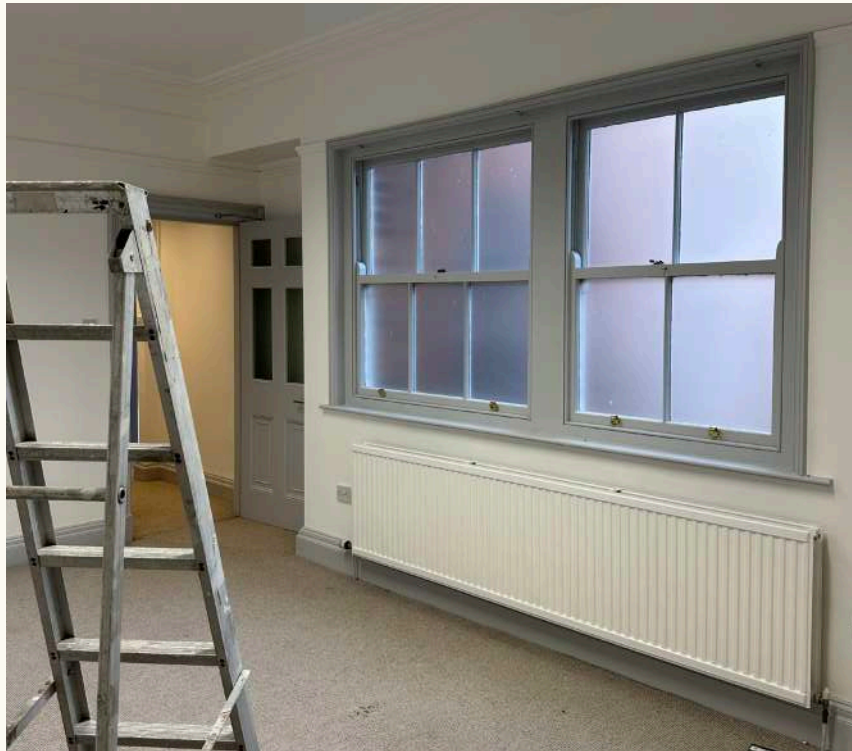
REF 13: FIRST FLOOR REAR SASH WINDOWS
