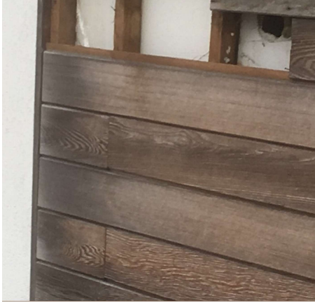
Existing timber cladding
