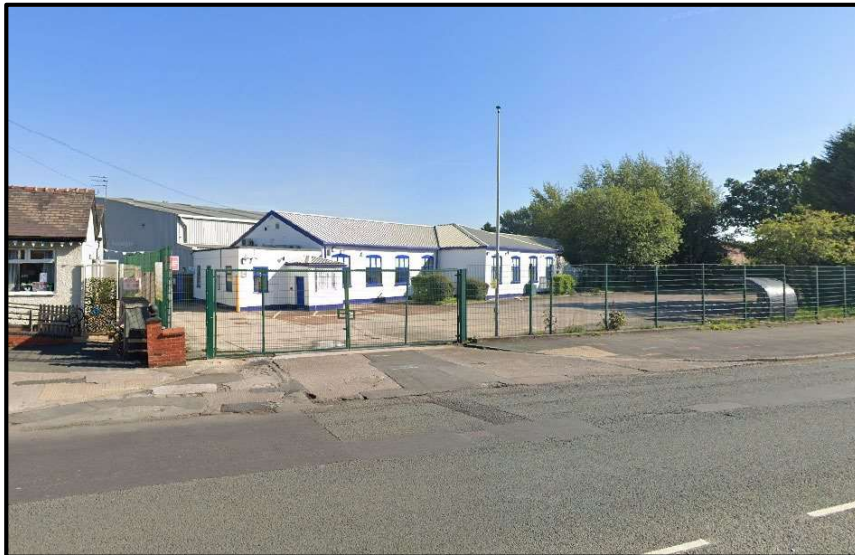
PHOTO 1: VIEW OF THE SITE FROM HOLLINWOOD AVENUE.
