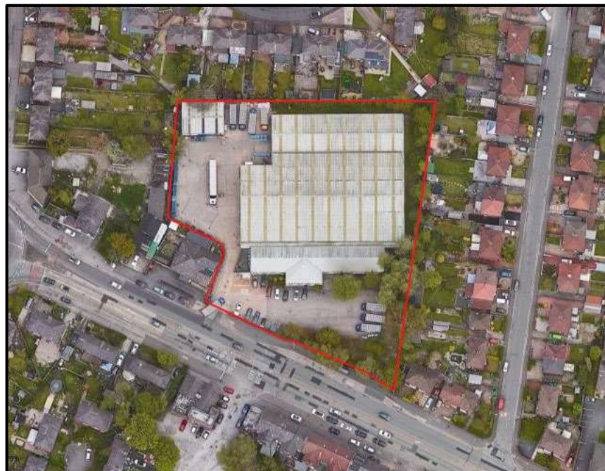
PHOTO 2: AERIAL VIEW OF THE SITE
