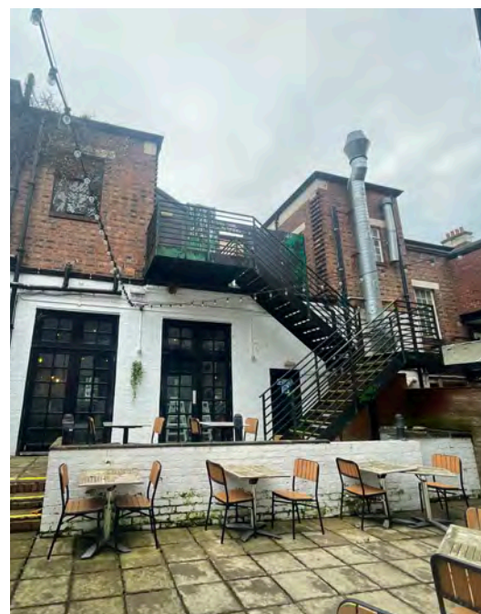
Photograph of rear external space
