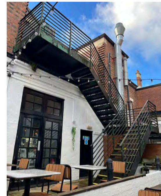
Photograph of rear external stair
