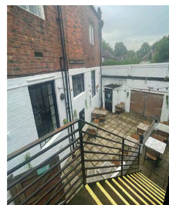
Photograph of rear external space
