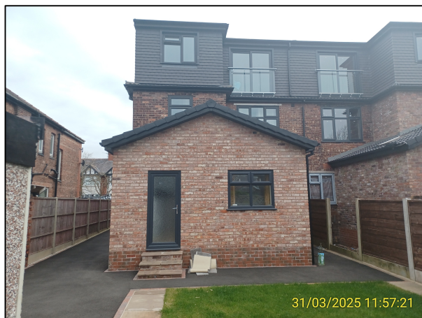
Photograph 1 Single Storey Rear Extension as built
