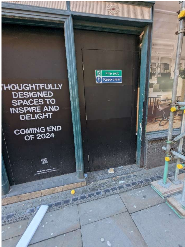
Figure 16- Current condition of main entry
