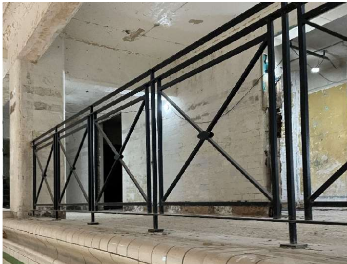
Figure 13- Existing balustrade on site
