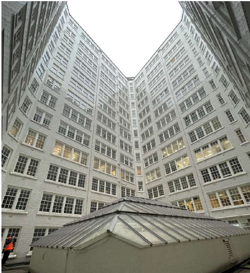
Figure 1- View of offices from internal void (Harrison Ince)
