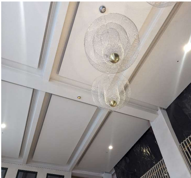
Figure 15- Acoustic panels and coffer detail in Sunlight House reception (separate works)
