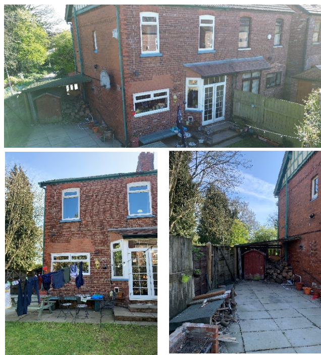
Rear and side of the property
