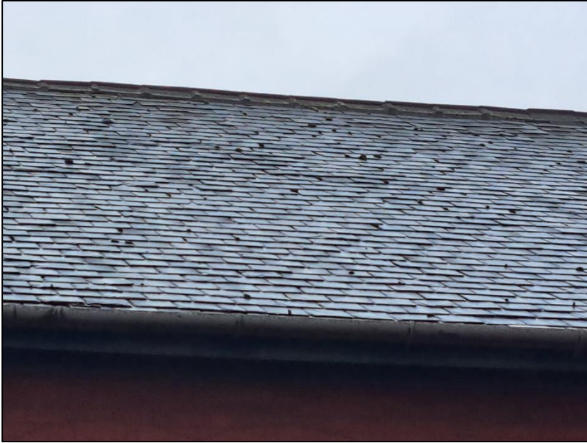
Photograph 5 showing the northeast elevation of the roof
