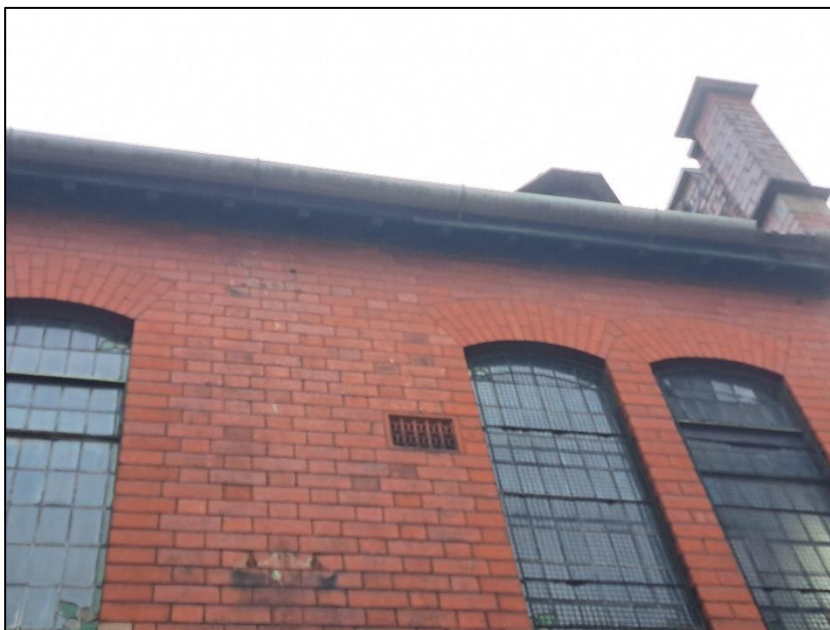
Photograph 2 showing the wooden facias of the building
