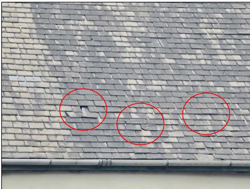
Photograph 4 showing part of the roof on the southwest elevation
