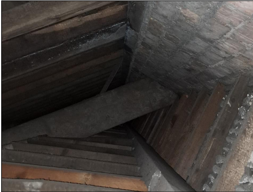
Photograph 11 showing a limited view of one side of the roof void
