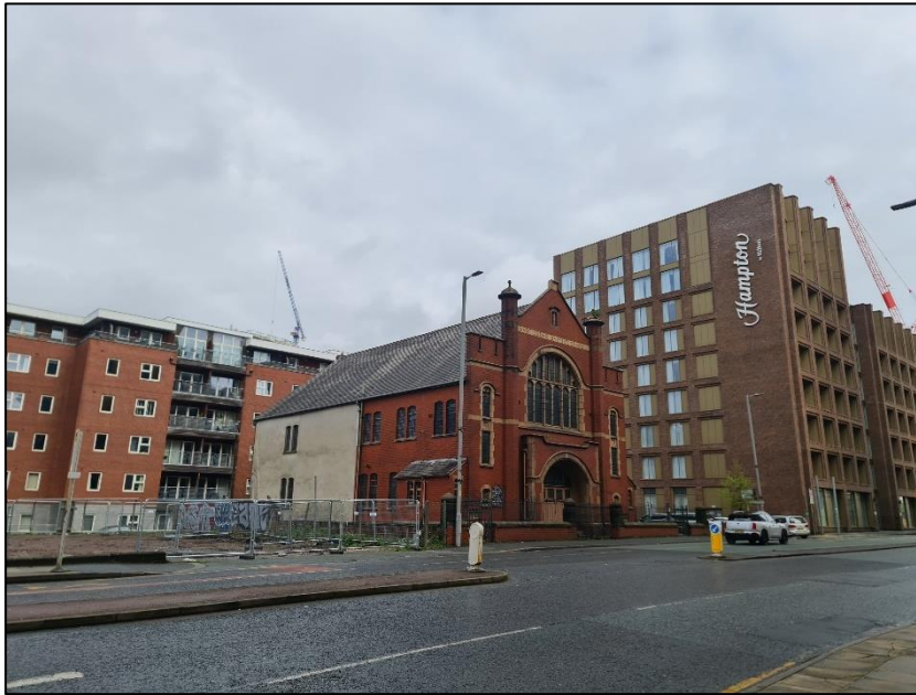
Photograph 1 showing the southwest elevations of the building
