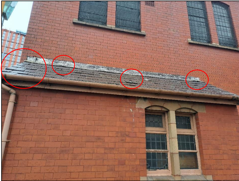
Photograph 7 showing the roof of the lean-to on the northeast elevation
