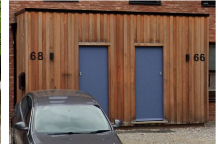
C: Entrance: Cedar Timber Cladding
