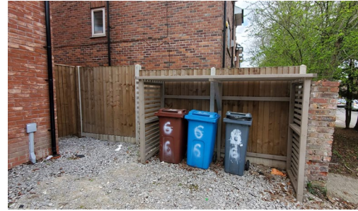
New Bin Storage - Cladded in Timber Latt
