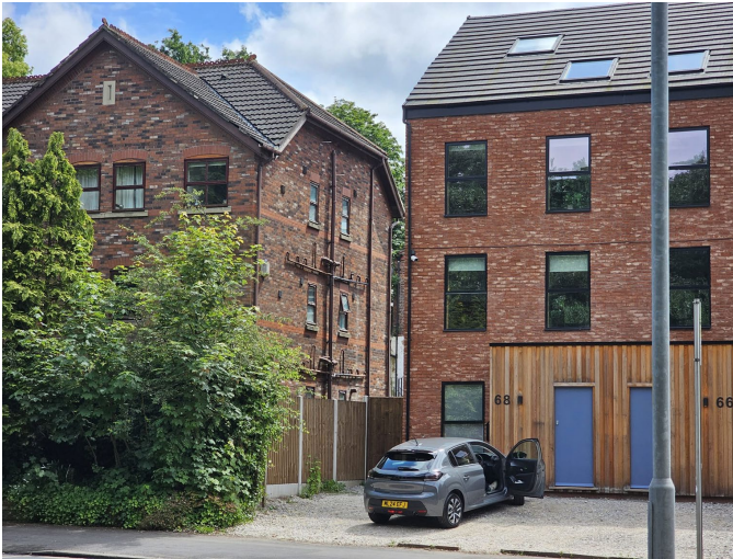
Access from the front, to the rear, restricted with a full height lockable gate
