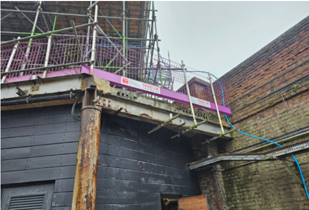
External photos of plant room, steel columns and beams have rusted due to water ingress issues.
