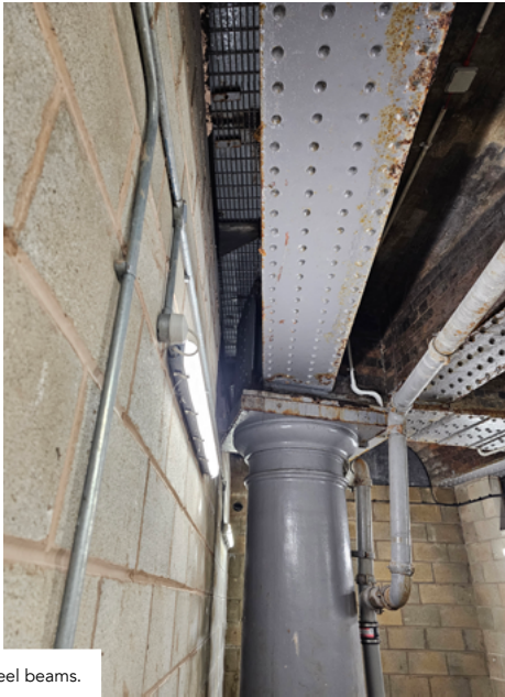
External photos of plant room, steel columns and beams have rusted due to water ingress issues.
