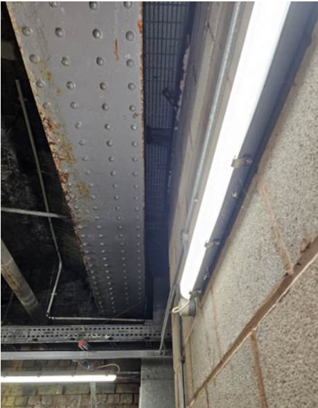
Internal photos of plant room, showing water ingress and rusted steel beams.
