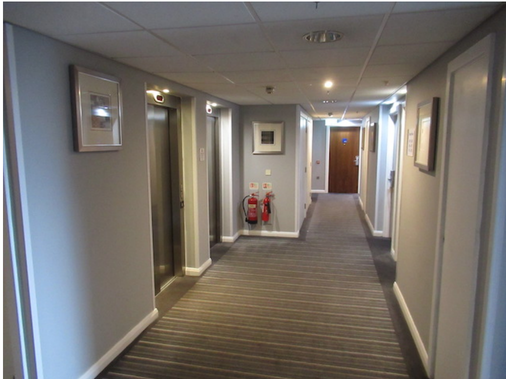
19. General view of finishes to lift lobbies / bedroom corridors
