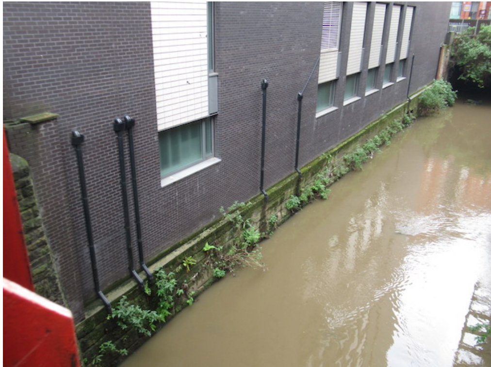
3. Basement and ground floor levels adjoining River Medlock
