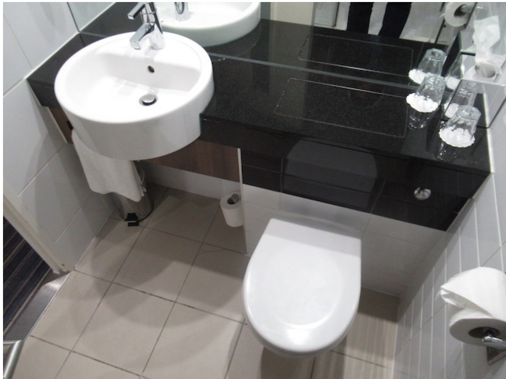
22. Typical condition of bathroom pod finishes
