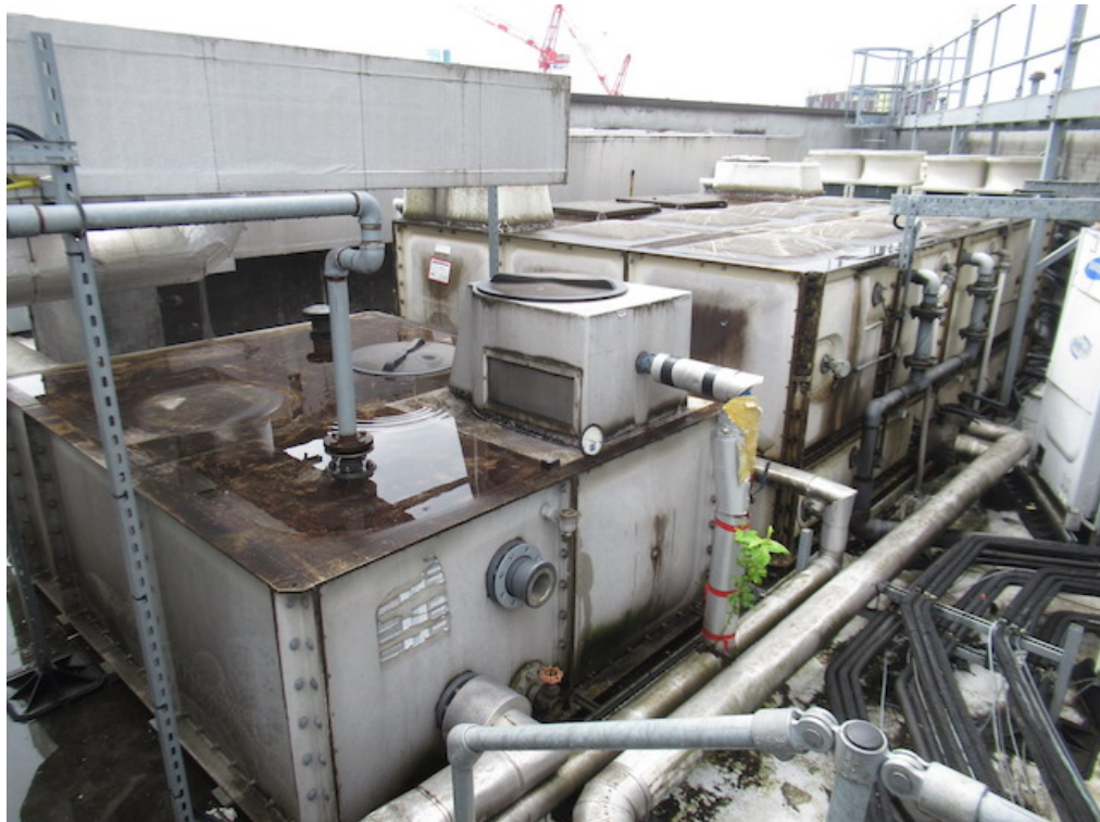
6. General view of water storage tanks to main roof
