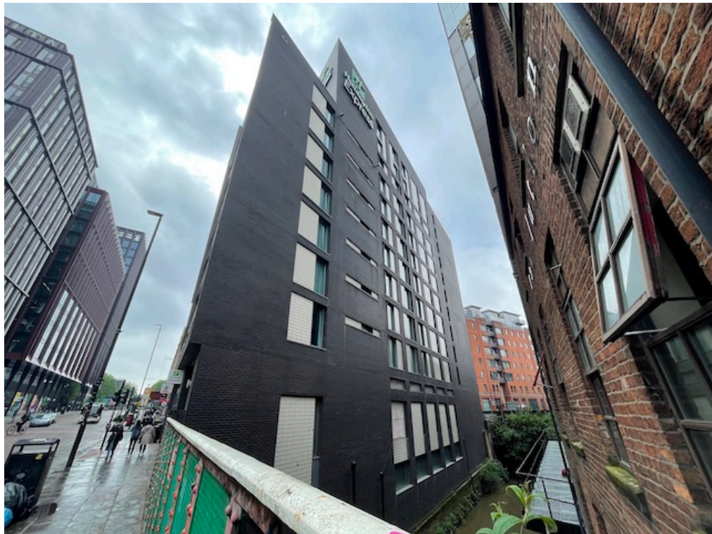
2. General view of north elevation facing onto River Medlock (from bridge)
