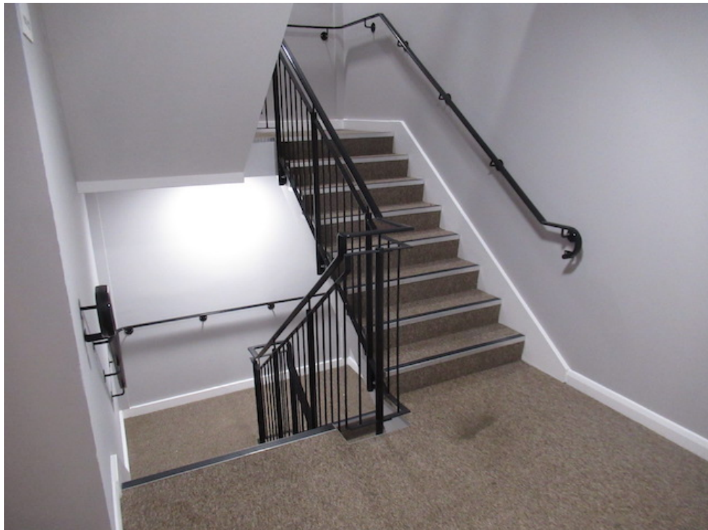
20. General view of circulation staircase finishes
