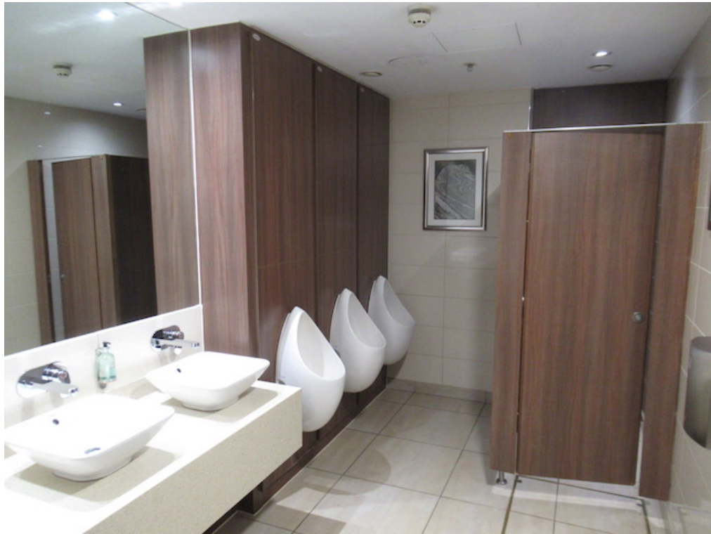
13. General fair condition of guest toilet finishes
