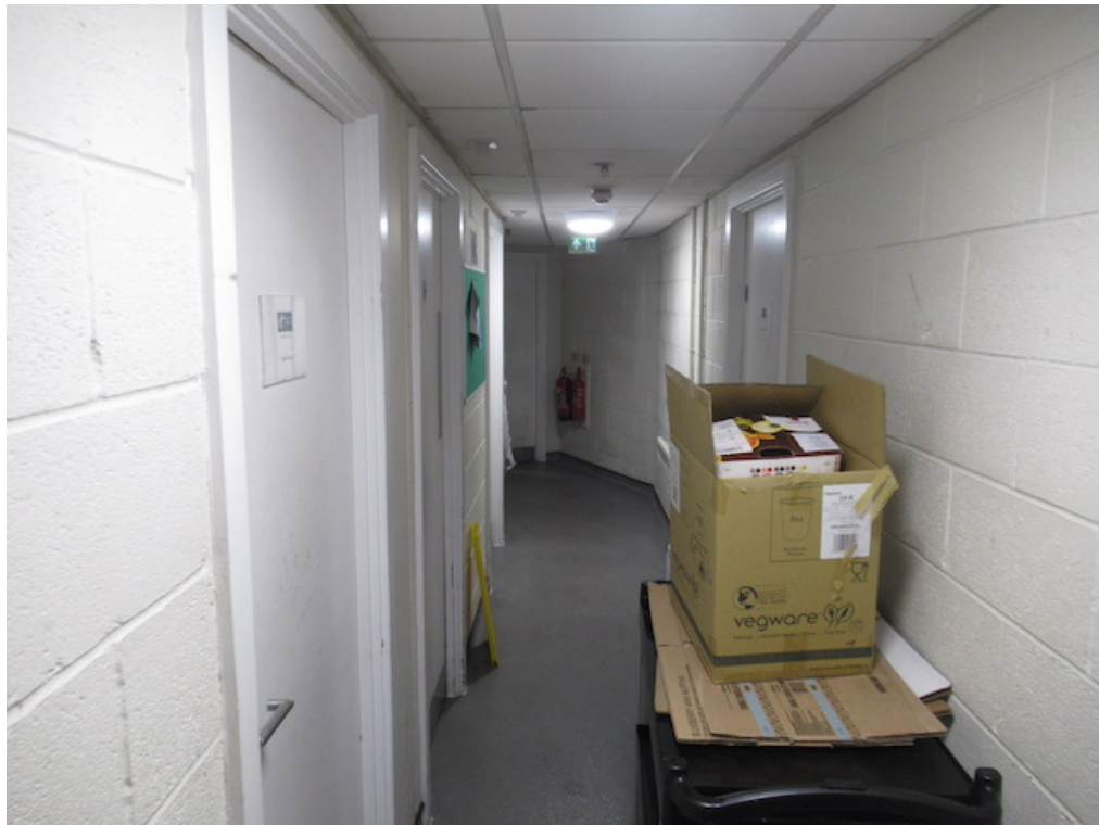
16. Typical worn finishes to 'back of house' staff area finishes
