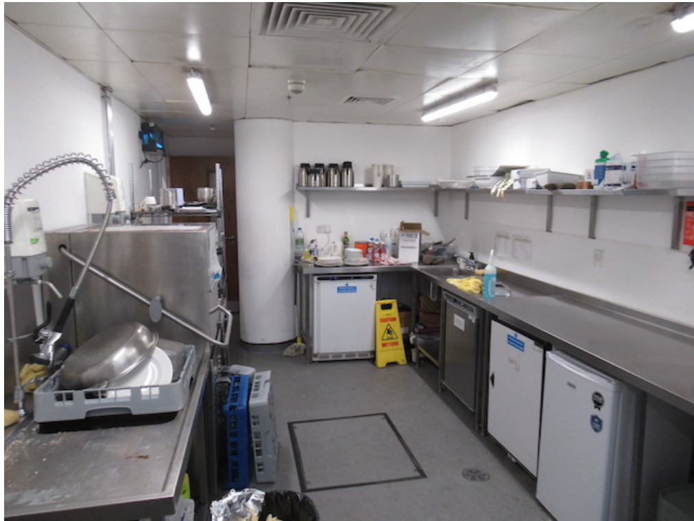
15. General view of kitchen finishes
