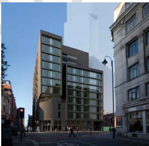
Figure 14 – The existing view of the building looking west. (Source: Stephenson Hamilton Risley STUDIO)
