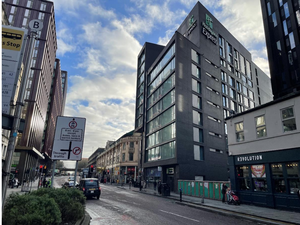
Figure 1a – Looking south-east along Oxford Street showing the Holiday Inn Express (The Site) to the centre right. (Source: SLHA January 2024)
