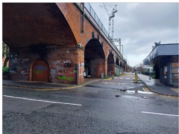
29. Altrincham Street and NR Viaduct, facing east
