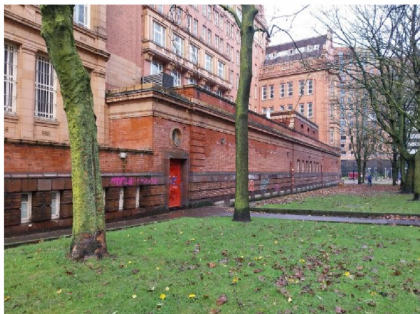
37. West of Sackville Street building, facing north
