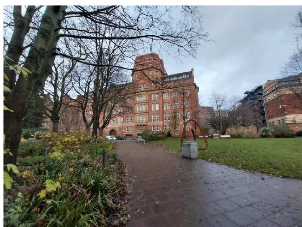
35. Sackville Street Building and gardens, facing north
