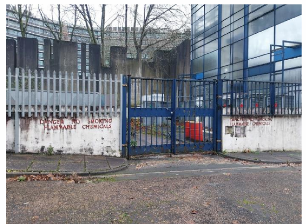
6. Flammable chemical storage area, north of Morton
