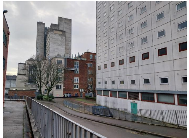
4. Rear of Wright Robinson and The Mill, facing south
