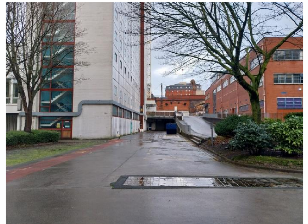
10. Rear of Wright Robinson, facing north
