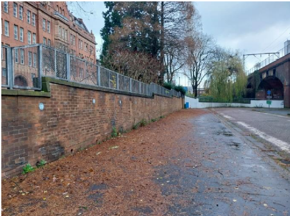
31. Vimto Gardens retaining wall, facing east
