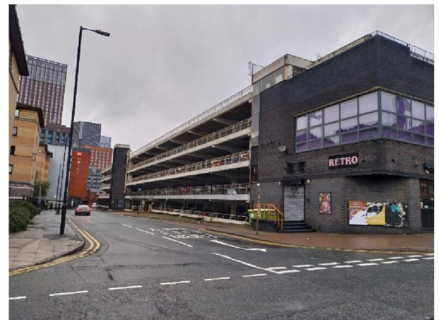
28. Charles Street Car Park, facing west
