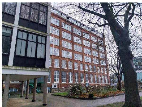
16. Western elevation of The Mill, facing southeast
