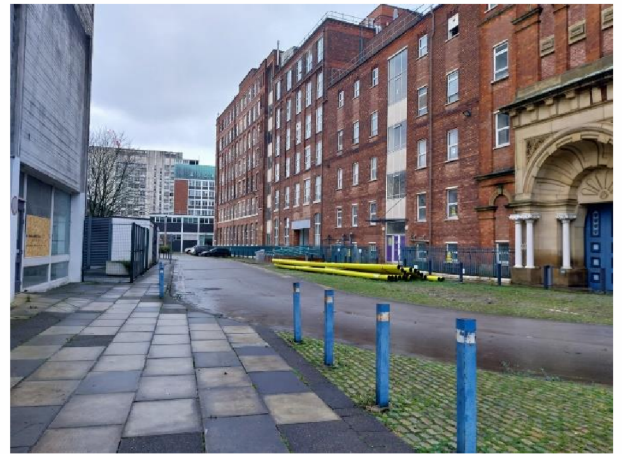
8. Front of The Mill and Service Road, facing west
