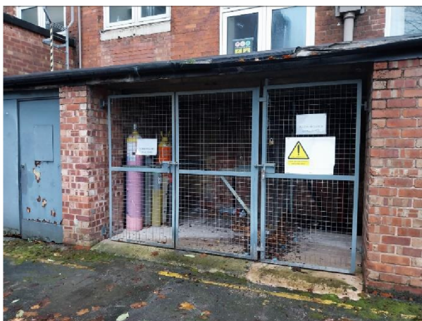
11. Liquid gas storage cage at The Mill, facing west
