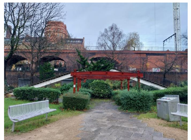
12. Butterfly Staircase, facing north
