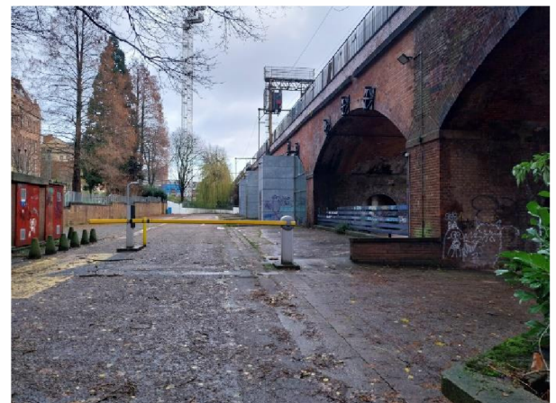
30. Car Park and gas governor, to north of NR Viaduct, facing east
