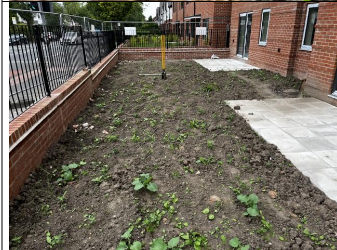
Photograph 17: View showing soft landscaping area surrounding the apartment block (area 6).
