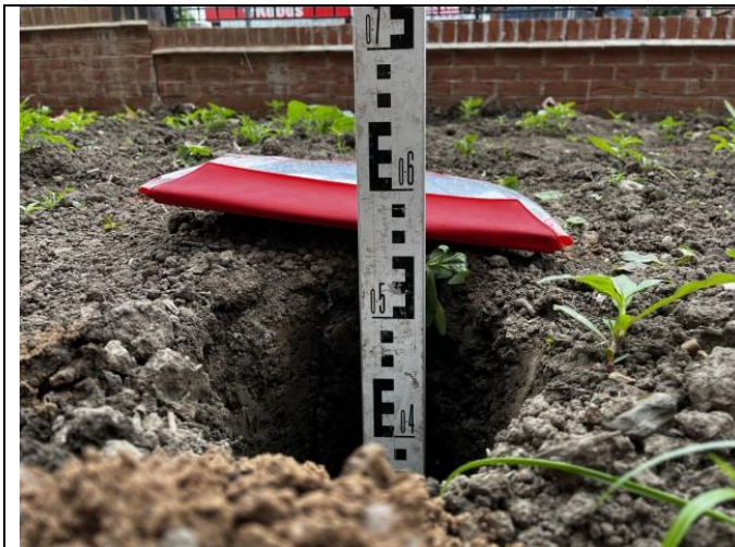
Photograph 16: Evidence of suitably chemically validated topsoil with a minimum of 150mm growing medium in the soft landscaping area surrounding the apartment block (area 6) over geotextile membrane.
