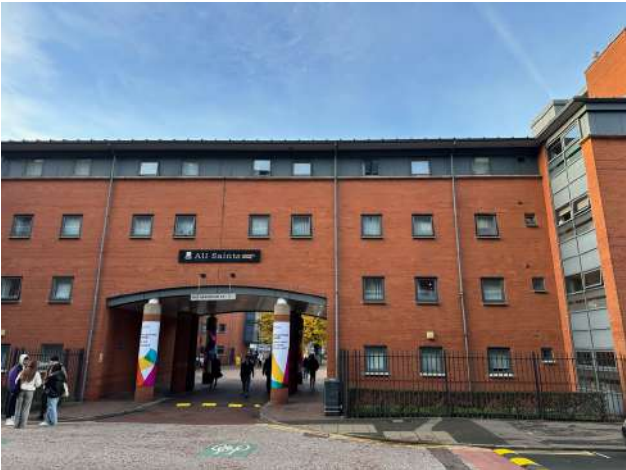
Plate 8: Entrance to building
