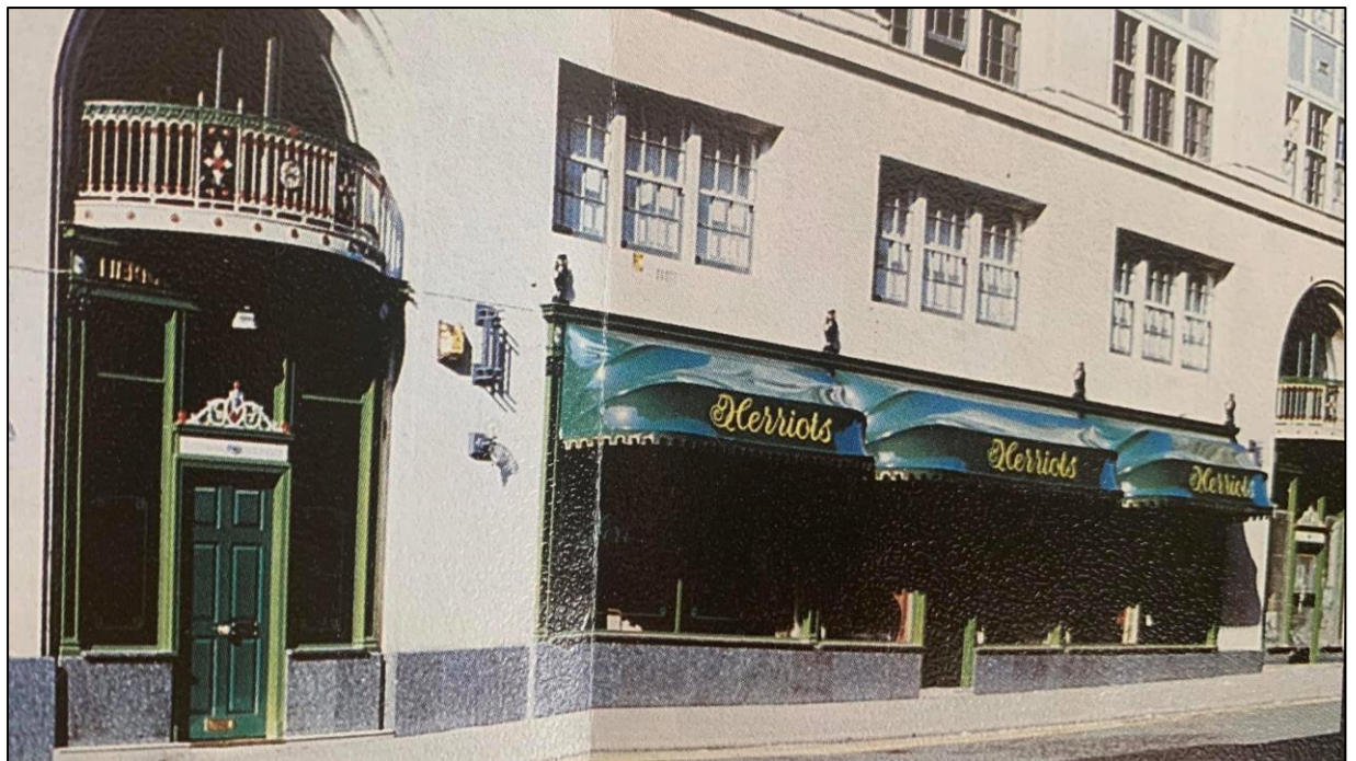
Figure 16 – 1980's image of Quay Street elevation, showing canopies above the window openings with Herriots lettering, as well as the paint scheme to the metalwork which exists today.
