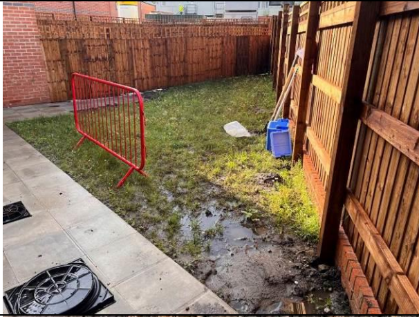
Photograph 18: View showing rear garden (Plot 12).
