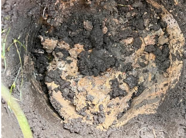
Photograph 19: Evidence of suitably chemically validated topsoil with a minimum of 150mm growing medium in garden areas (Plot 12).
