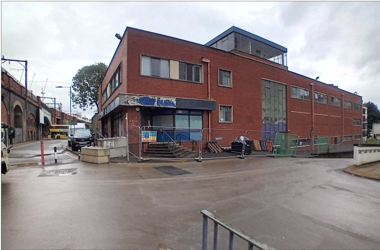
Plate 9: Moffat Building, looking east.
