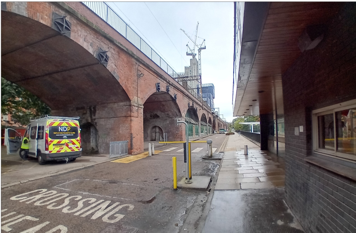
Plate 4: Altrincham Street East, looking east from the Gatehouse.
