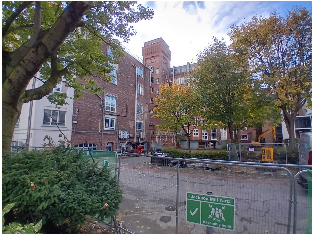
Plate 12: Looking south west - earlier section of mill visible with distinct arched windows.
