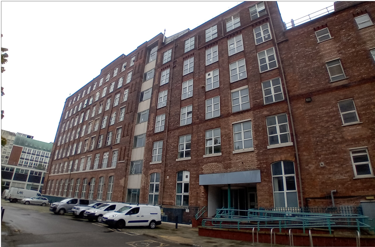
Plate 13: Jackson Street Mill, west end, looking north.
