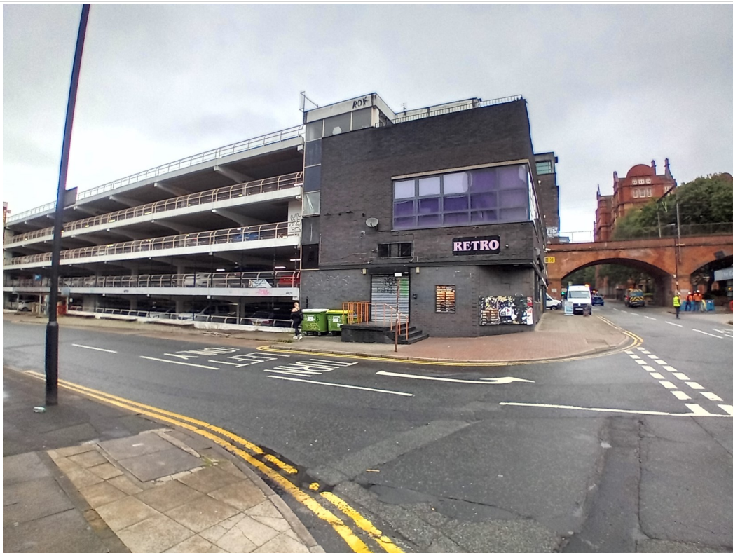
Plate 14: Charles Street Car Park, looking north.
