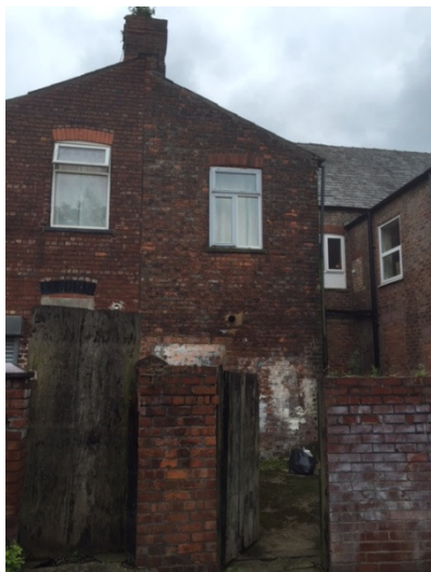
Rear Elevation to Application Property.
