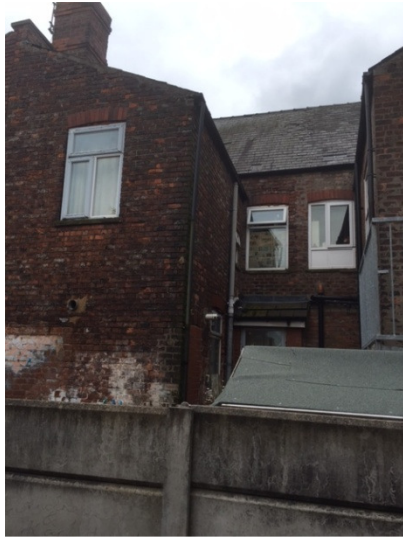
Rear Elevation to Application Property.
