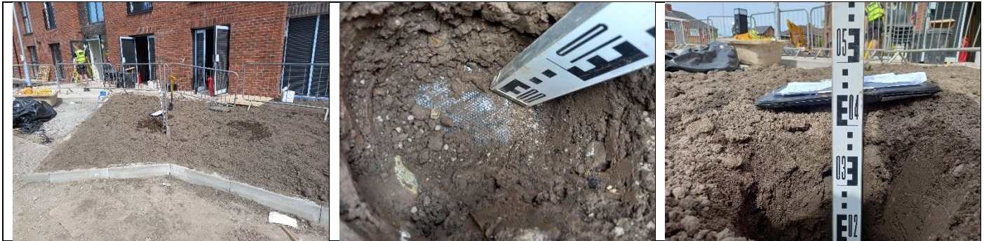
View of membrane and soil in capping layer excavation in landscaped Area 8.
