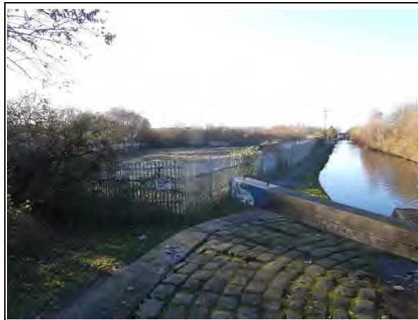
Looking Southwesterly Towards the Site from Lock No. 14
