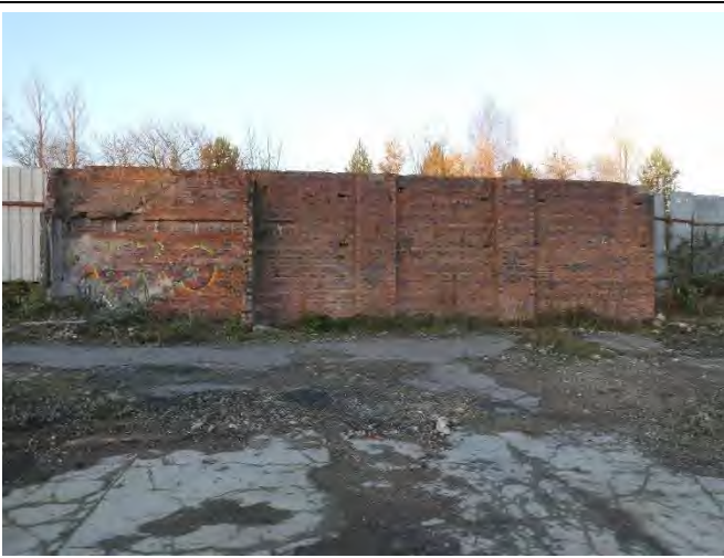
High Brick Walling with Buttresses
