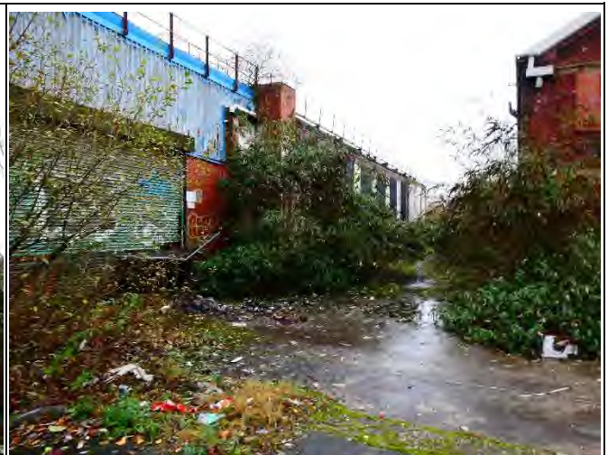
East Elevation of Area 13
