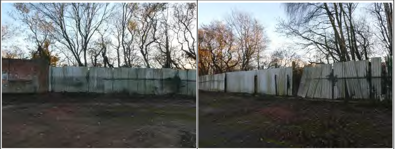
Metal Sheetting and Concrete Posts
