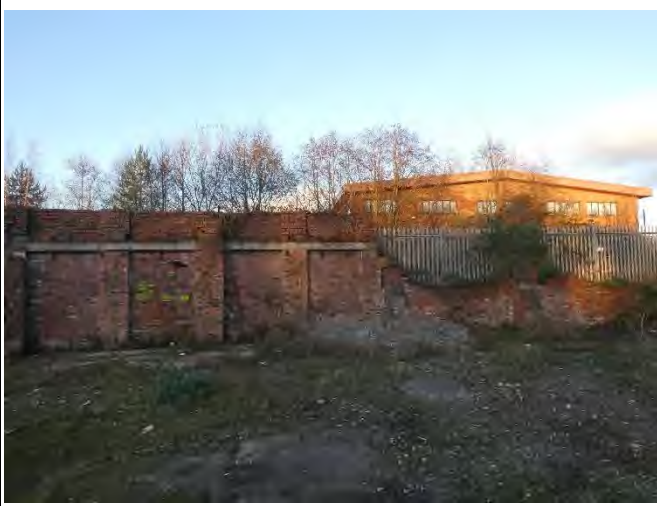
Eastern End of the Northern Wall with Buttresses
