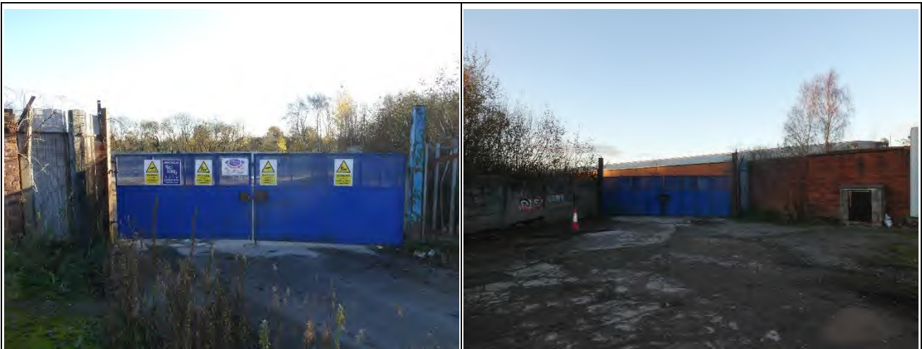
Metal Entrance Gates to the North Along Towpath
