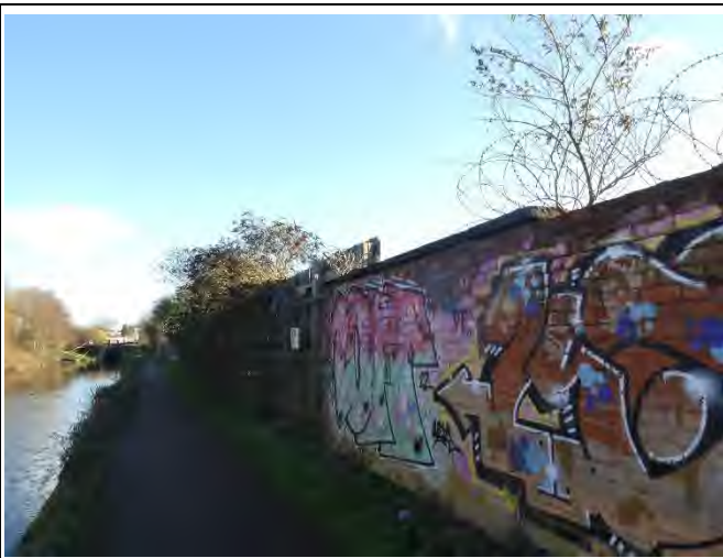
Boundary Wall and Metal Security Fence Adjacent to Canal Lock Fourteen
