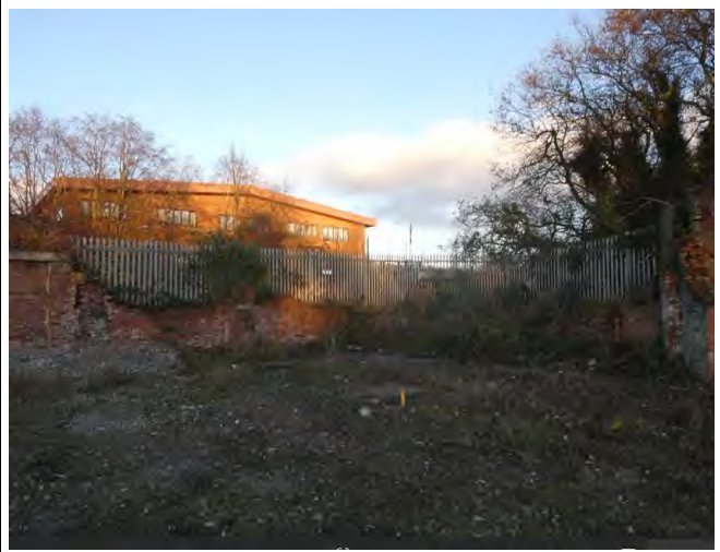
Partial Walling and Metal Security Fencing at the Northeast Corner, Lock 14 Beyond
