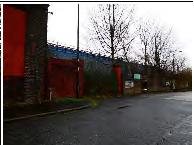
West Boundary Along Crabtree Lane
