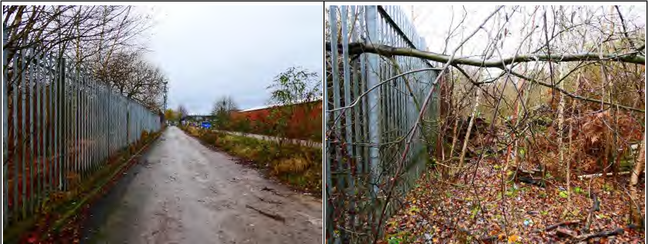
North Boundary Metal Security Fencing Looking West Along the Towpath of Ashton Canal
