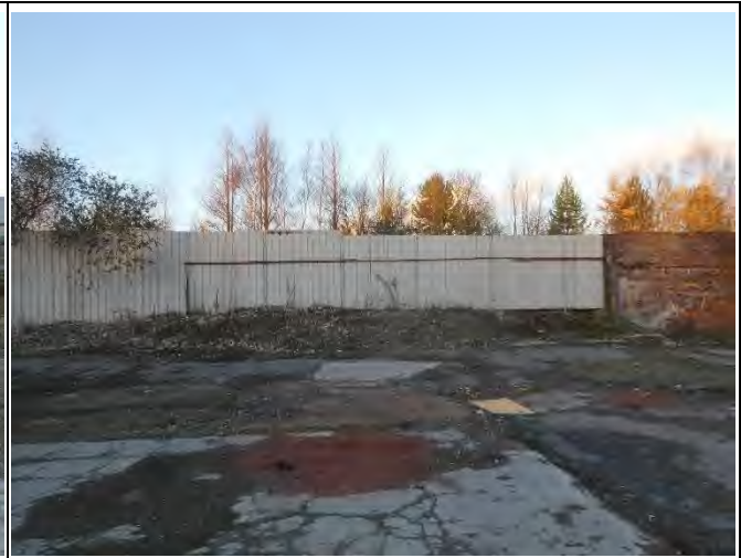
Metal Sheetting/Metal Security Fencing
