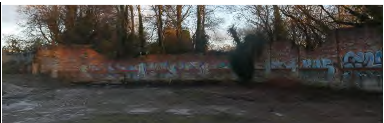
Brick Walling with Buttresses
