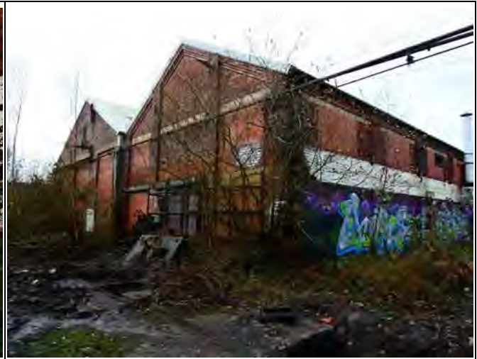
North Elevation of Area 8
