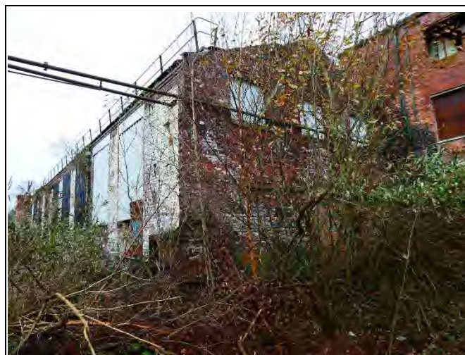
North Elevation of Area 13
