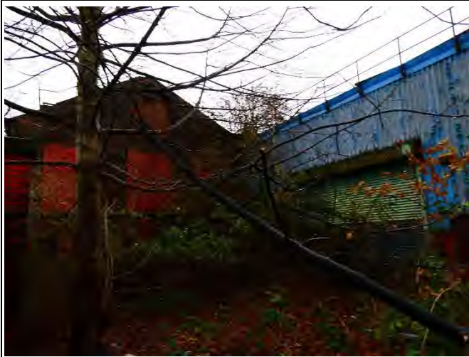
South Elevation and West Elevation of Area 13
