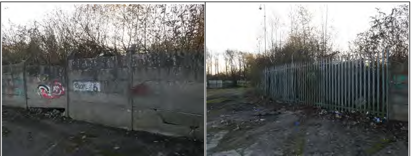
Boundary at the Extant Buildings, Consisting of Concrete Blocks and Metal Security Fencing
