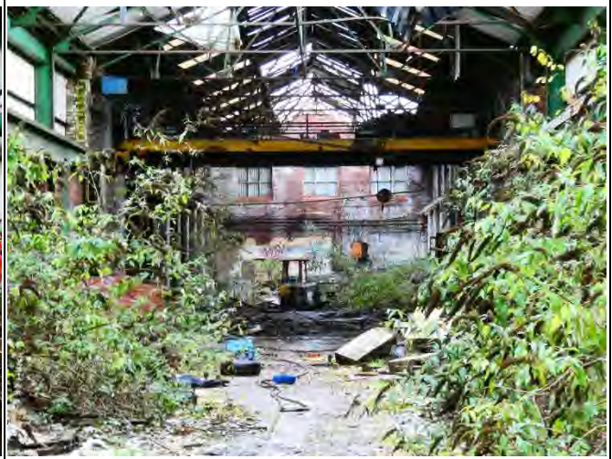
Remnants of an Overhead Crane
