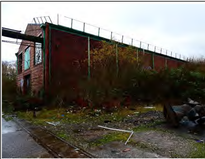
North and West Elevation of Area 16
