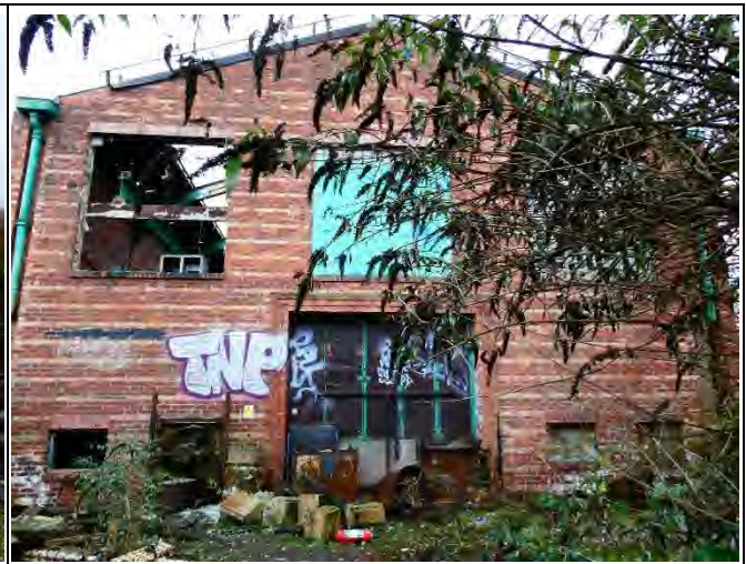
North Elevation of Area 16
