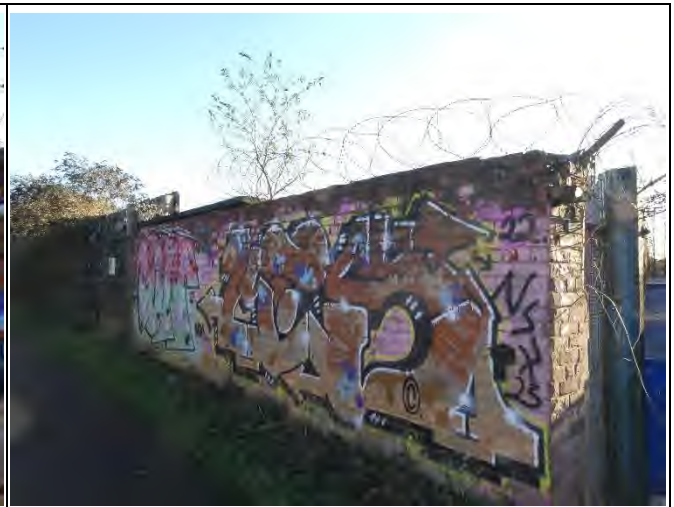
Boundary Wall Adjacent to the Access at the Towpath
