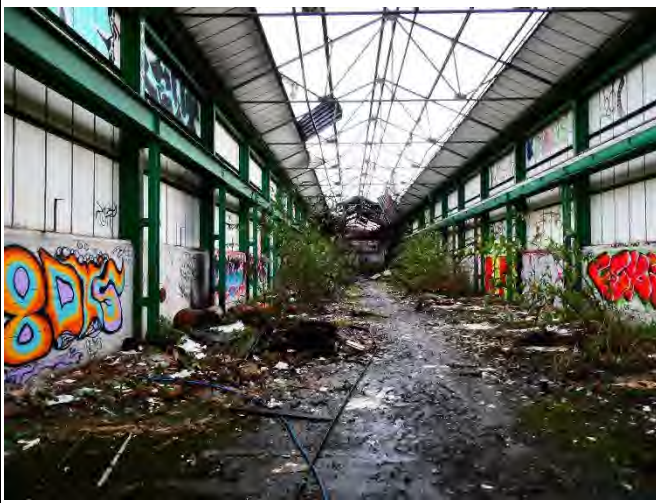
Semi-Derelict Interior of Area 13
