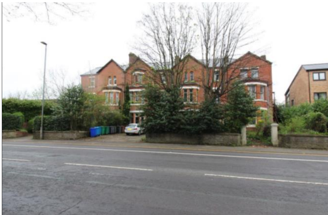
View of application property frontage (Bury Old Rd)
