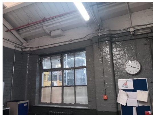
Figure 17: The window to the Engineer's Area kitchen is proposed to be refurbished. Source: SLHA 2024
