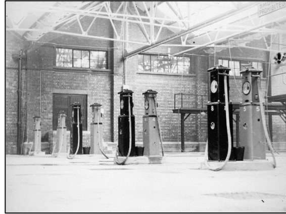
Figure 21: 1937 photograph of the petrol and fuel pumps within the Bus Depot that catered for the buses used for public transport. Source: Transport Department, Greater Manchester Lives Archive
