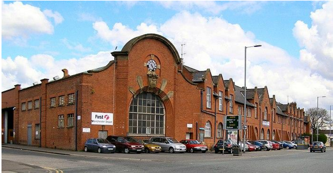
Figure 3: View of the Bus Depot from the corner of Boyle Street and Queens Rd. Source: Google Maps.
