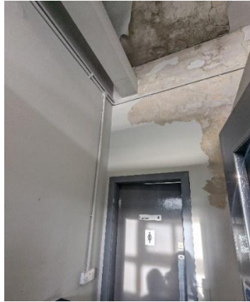
Figure 12: The ceiling finishes to the Driver's Area have been damaged by water penetration issues at roof level. Source: SLHA 2024
