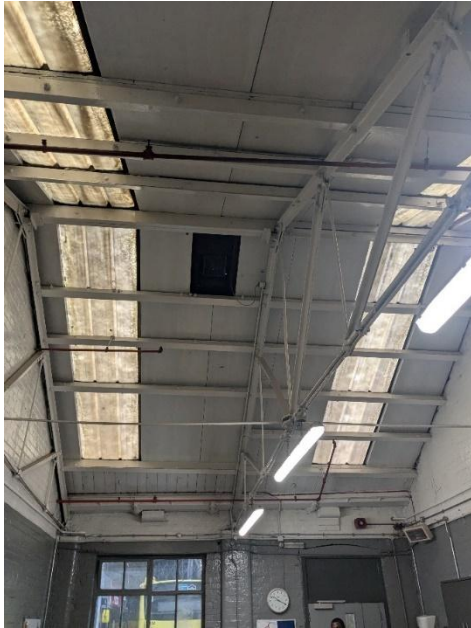
Figure 6: Original steel trusses are extant throughout the building. Proposals include installing suspended ceilings in selected areas, concealing the historic trusses. Source: SLHA 2024
