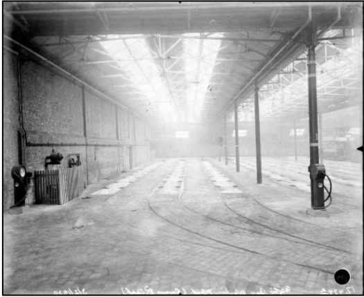
Figure 20: 1930 photograph of the Bus washing plant within Queens Road Bus Depot. This was built to support the influx of motorbuses that Manchester Corporation had acquired. Source: City Engineers Department, Greater Manchester Lives Archive
