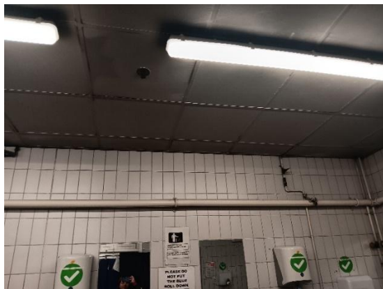
Figure 10: Modern suspended ceiling grid and modern light fixtures, to be removed and replaced under the current Proposals. Source: SLHA 2024
