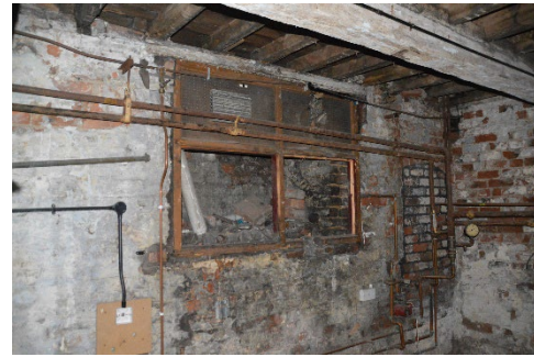
Existing basement photos of rear office with existing rotten window being replaced to match existing
