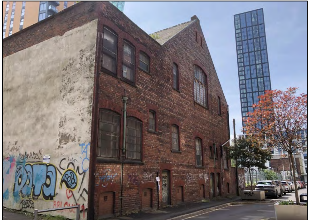
Plate 2 View of the northern and western elevations of the Baptist Church
