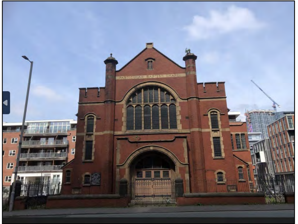
Plate 1 View of the eastern elevation of the Baptist Church
