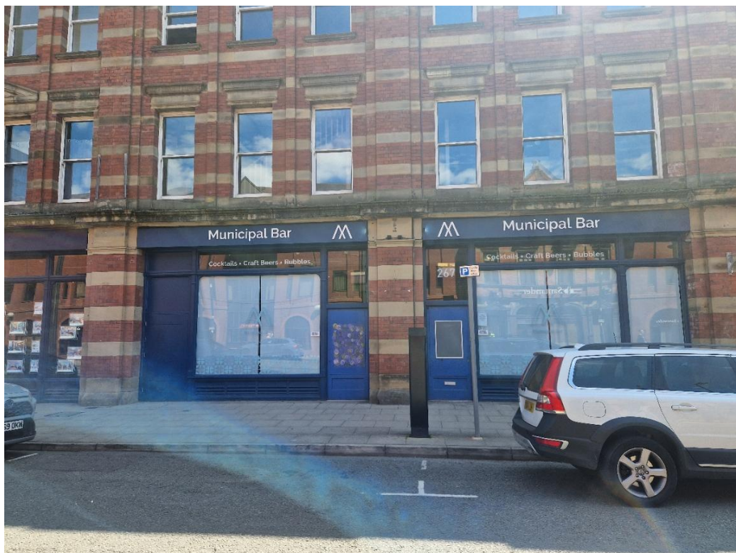
Image 4: Present Shopfront Elevation, Deansgate, Manchester
