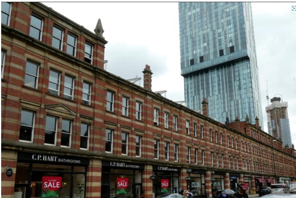
Image 2. Historic South view of Facade of shops and offices on Deansgate, Manchester Phil Platt 16 November 2018
