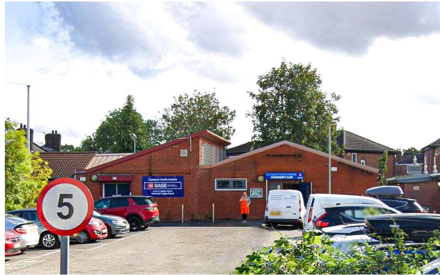
2. Front of building
