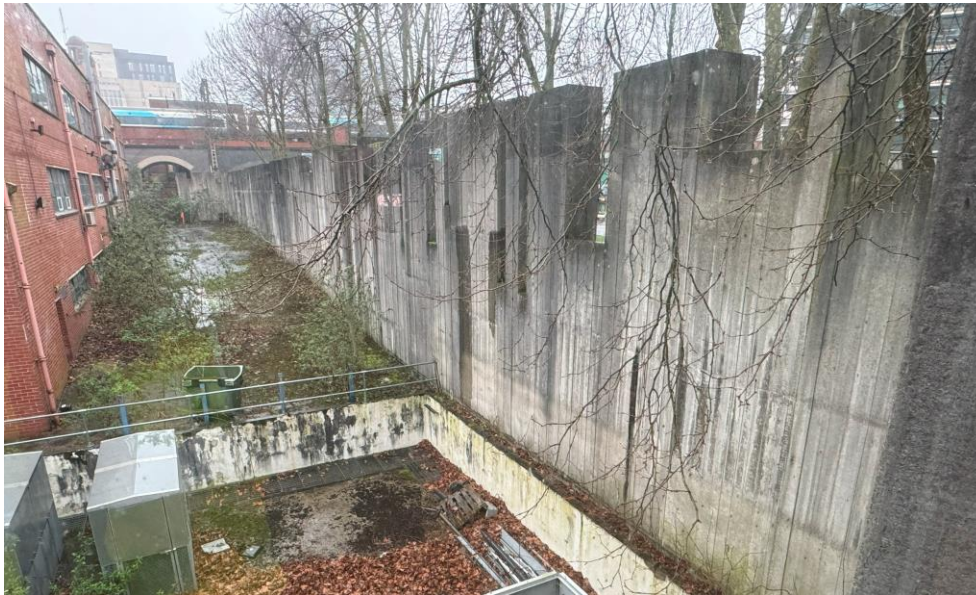
Figure 14: Image taken from inside the Morton Laboratory building
