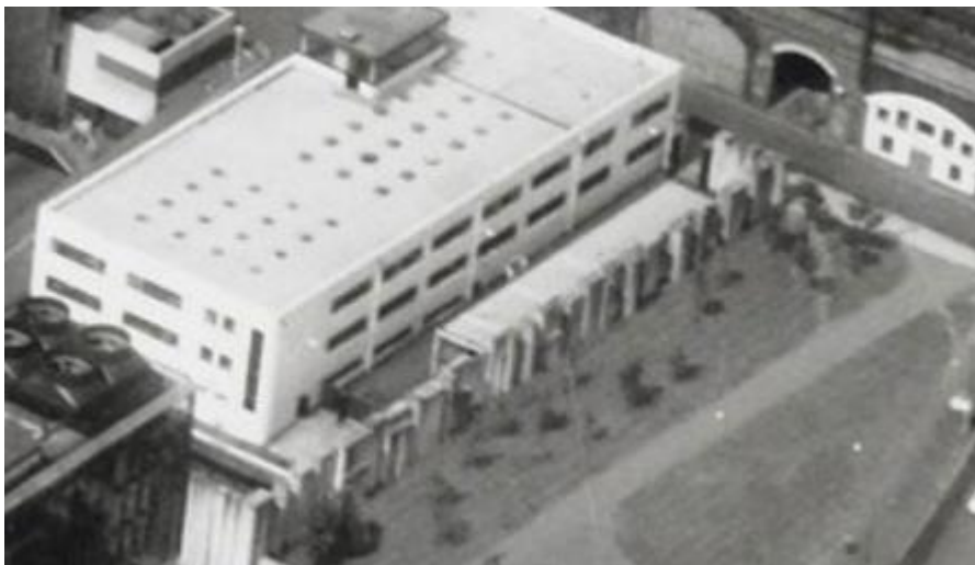
Figure 3: 1973 aerial image, close range of Hollaway Wall, featuring a single-storey lean-to behind. The Moffat building is extended and painted white. Source: Manchester Image archive.
