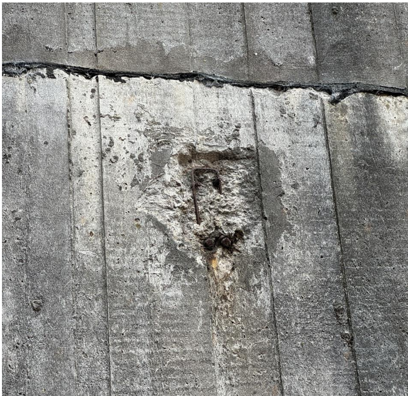
Figure 22: Remnants of former steel canopy structure (2024)
