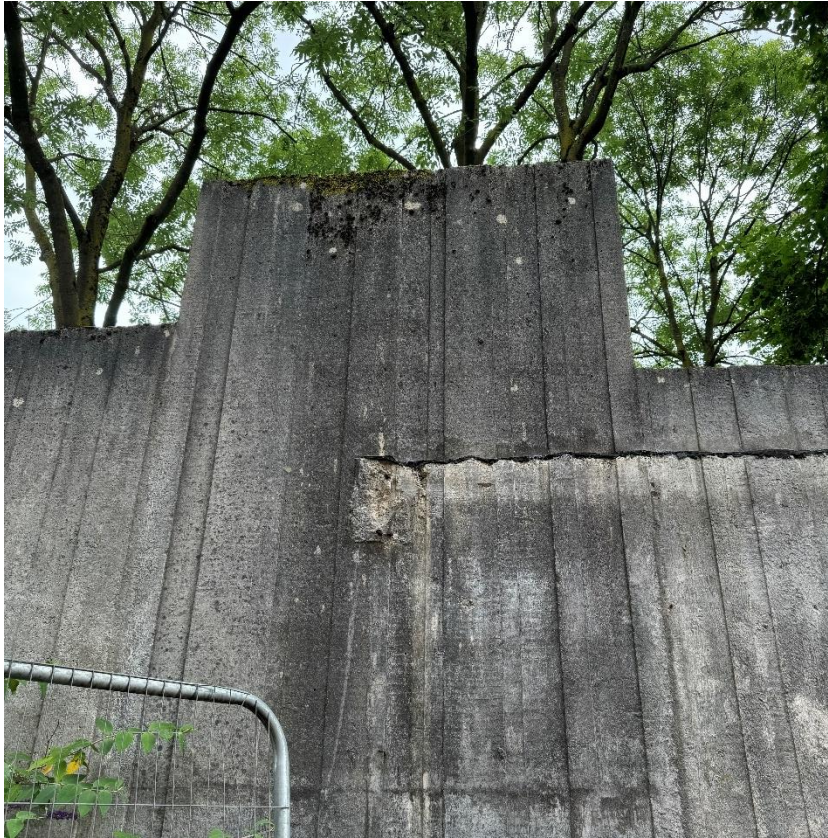
Figure 21: Evidence of former canopy structure (2024)
