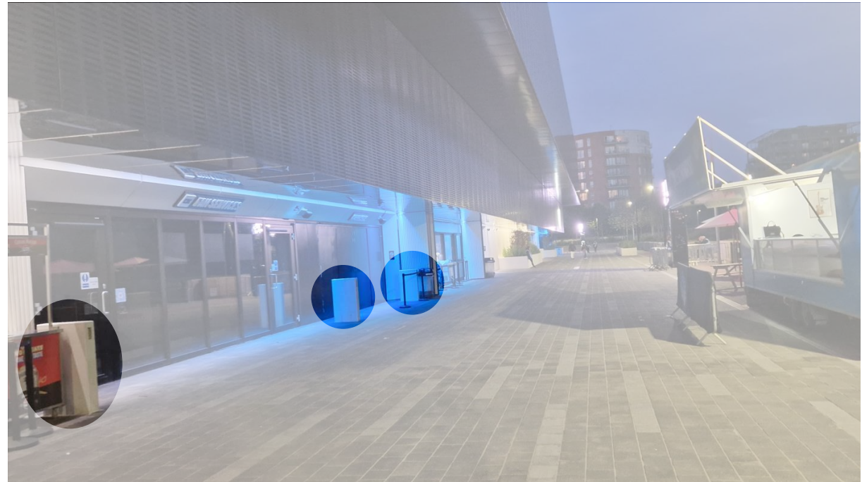
Existing concrete doorstops, 20 May 2025
