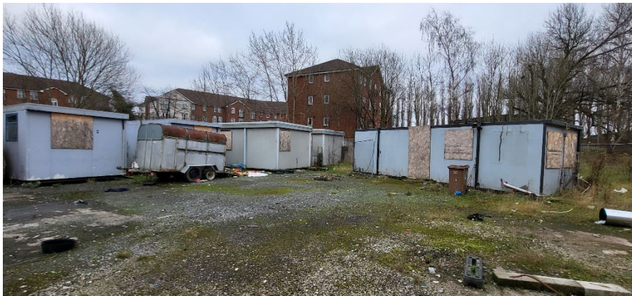
FIGURE 14 PORTACABINS ON SITE
