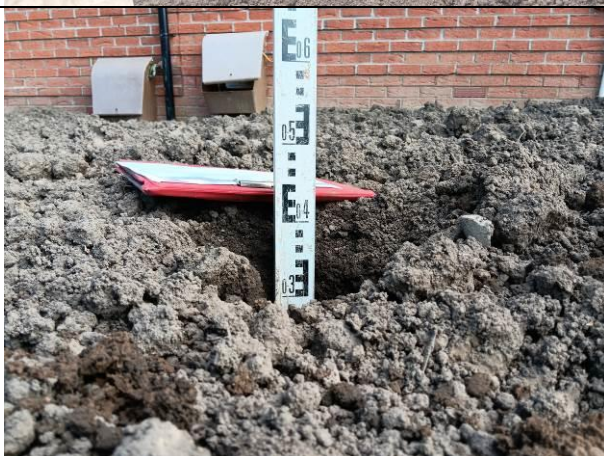
Photograph 4: Evidence of suitably chemically validated topsoil with a minimum of 150mm growing medium in front garden area (Plot 3) over natural strata.
