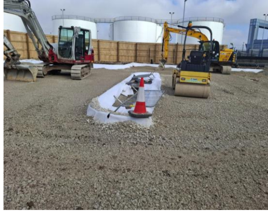
Install of type 3 sub-base
