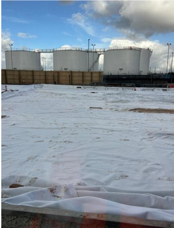
Install of top fleece
