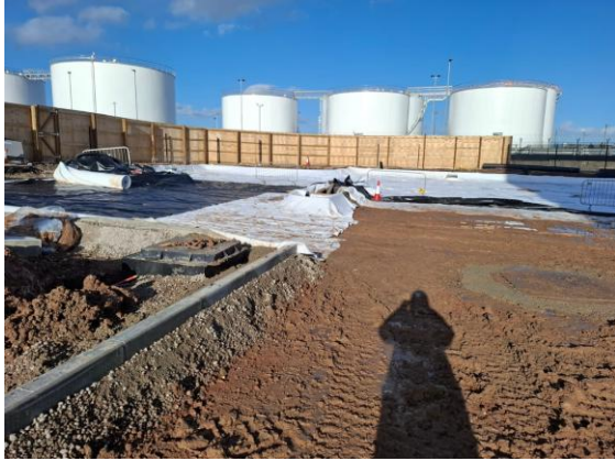
Install of membrane/fleece
