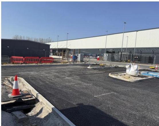
Install of porous binder course
