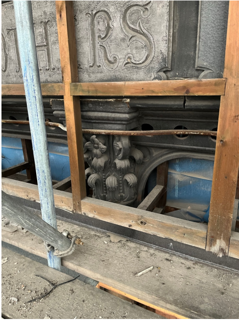
Column head and spandrel, with stone signage panels over.
