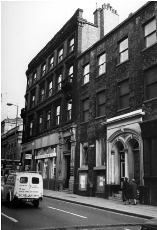
Photograph from 1973 with the traditional shopfront covered/removed.
