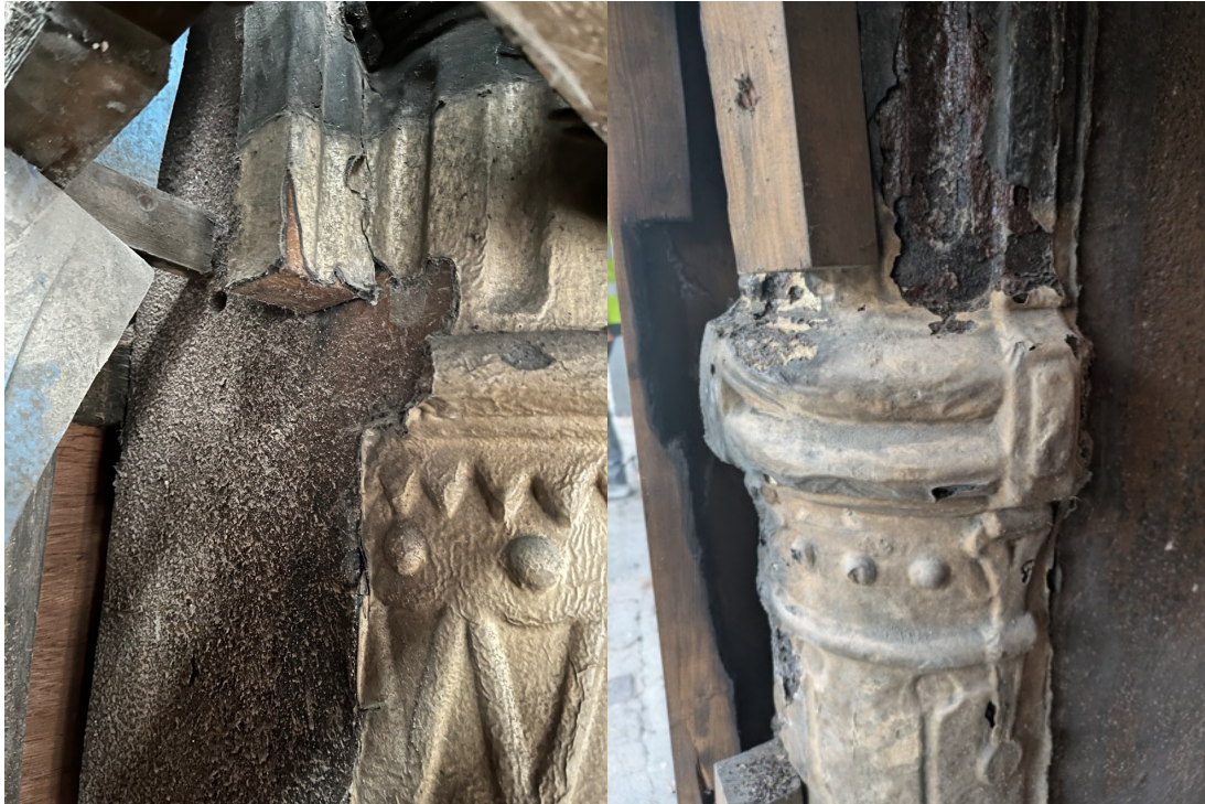
Side of cast iron column showing interface with later steel 'U' column.
