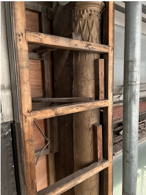
Main column body with the remaining aluminium modern shopfront visible to each side.
