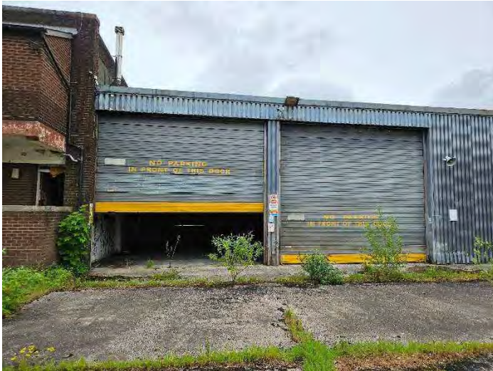
Photograph 11 – A view of the southern elevation of the building with access to the vehicle maintenance area.
