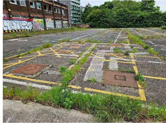
Photograph 2 – A view of the buied tank farm in the western area of the site.
