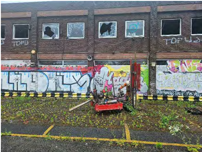
Photograph 15 – A view of the rig on position WS04.
