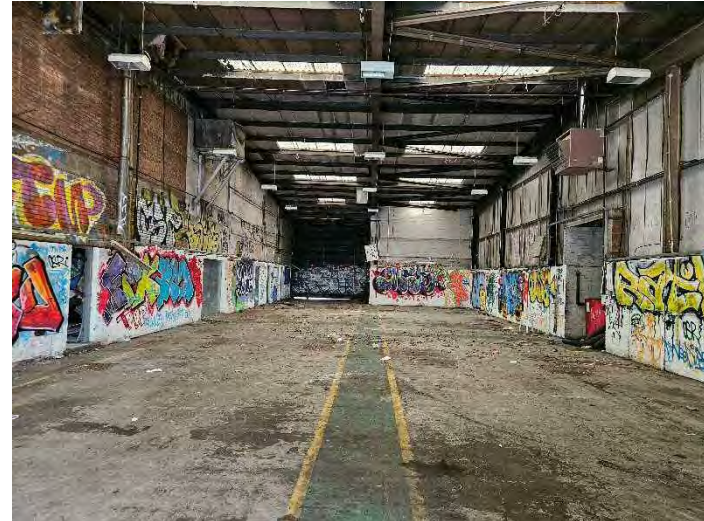
Photograph 12 – A view internally of the vehicle maintenance area.
