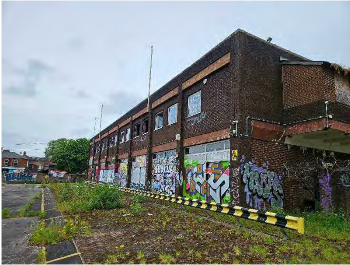
Photograph 1 – A view of the western elevation of the former bus garage building.
