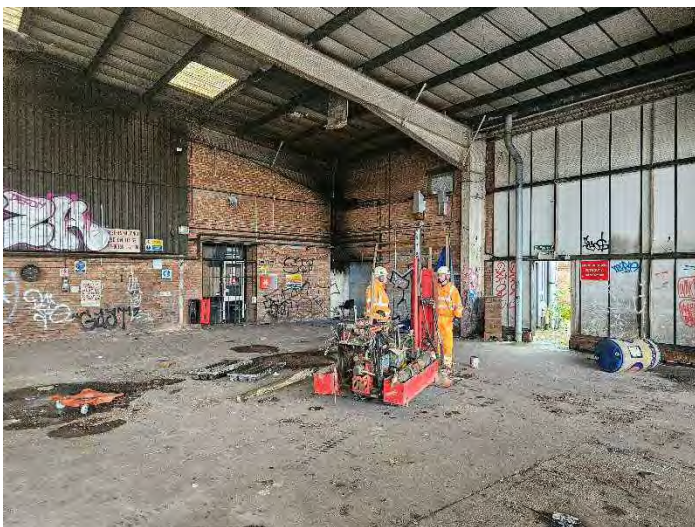
Photograph 17 – A view of the rig on position WS07.
