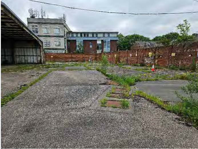
Photograph 9 – A view of the interceptors in the eastern external hardstanding area.
