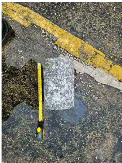
Photograph 19 – A typical example of the cored concrete hardstanding.
