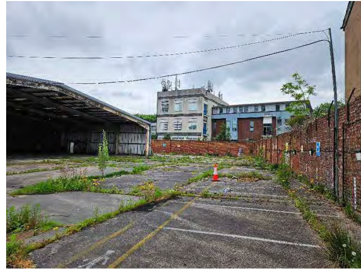
Photograph 6 – A view of the eastern external hardstanding area.
