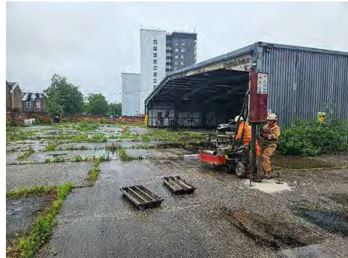
Photograph 16 – A view of the rig on position WS06.
