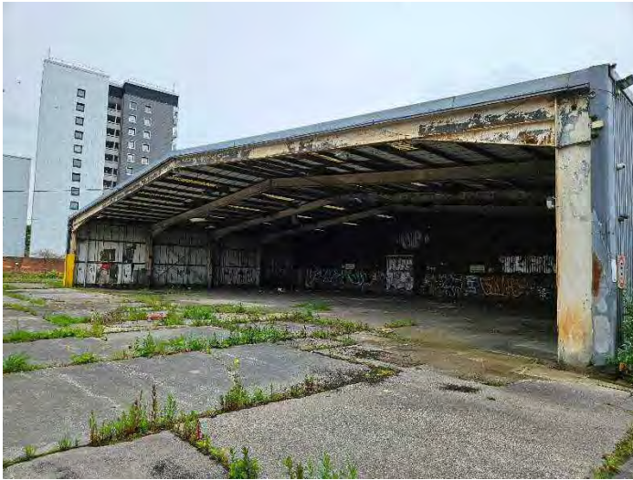
Photograph 5 – A view of the covered bus parking area in the east of the former bus garage building.
