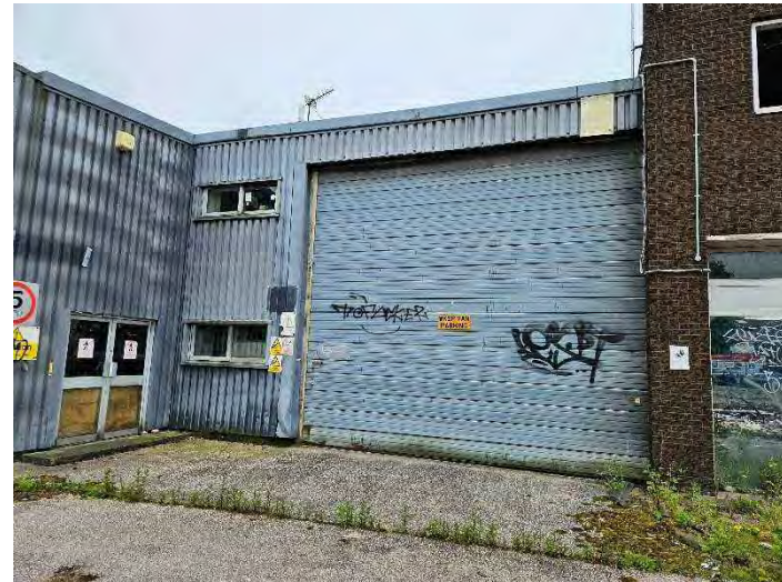
Photograph 4 – A view of the north elevation of the former bus garage building.
