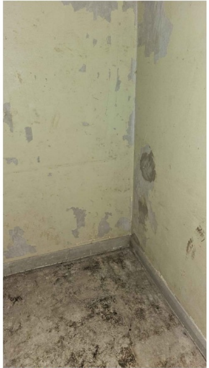
WALLS 9 -12 MODERN LINING
