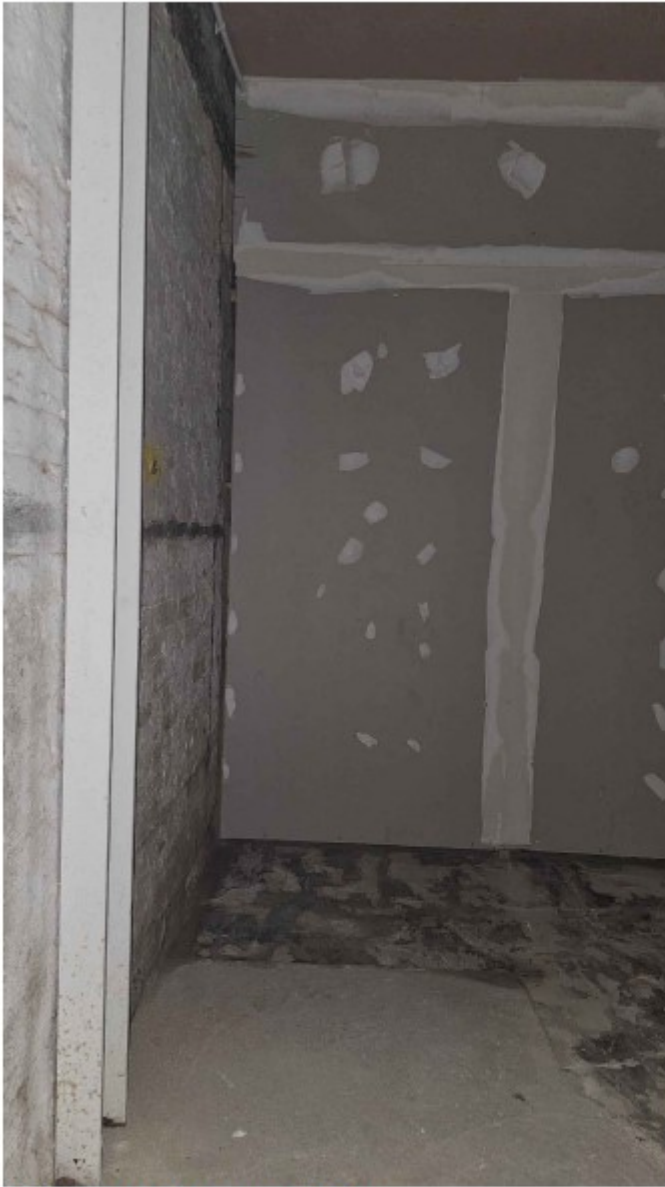
WALL 2 MODERN LINING PLASTERBOARD WALL 3 ORIGINAL FABRIC
