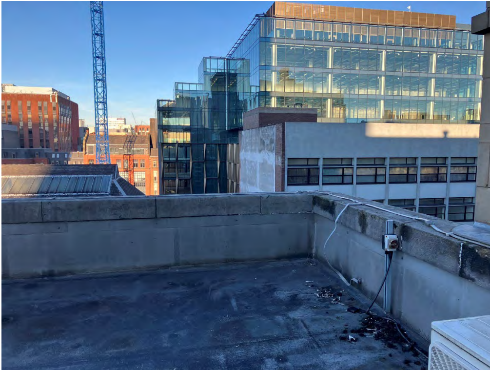
Plate 5. North facing view from the roof top
