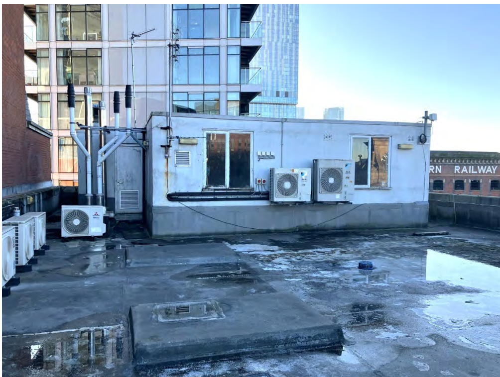
Plate 2 South facing view of the roof top plant room
