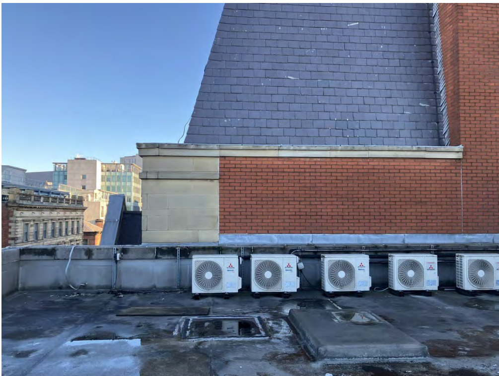
Plate 6. East facing view of the roof top
